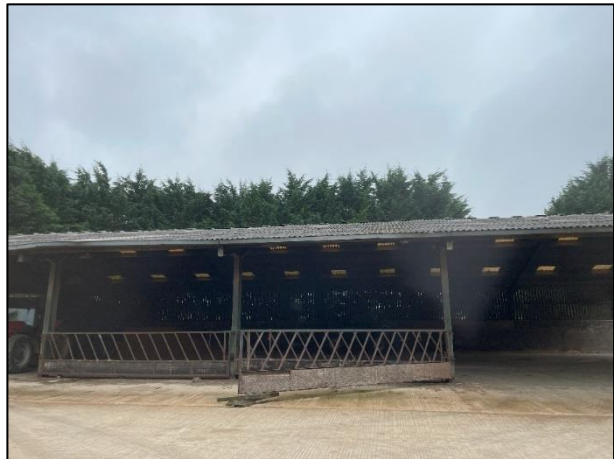
Photograph 10: Barn B1 north elevation. Image taken 14 th August 2024 by Charlene Watts.
