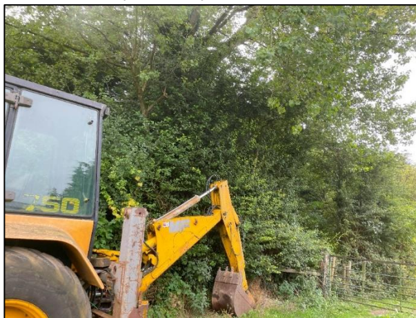
Photograph 4: Hedgerow H1. Image taken 14 th August 2024 by Charlene Watts.
