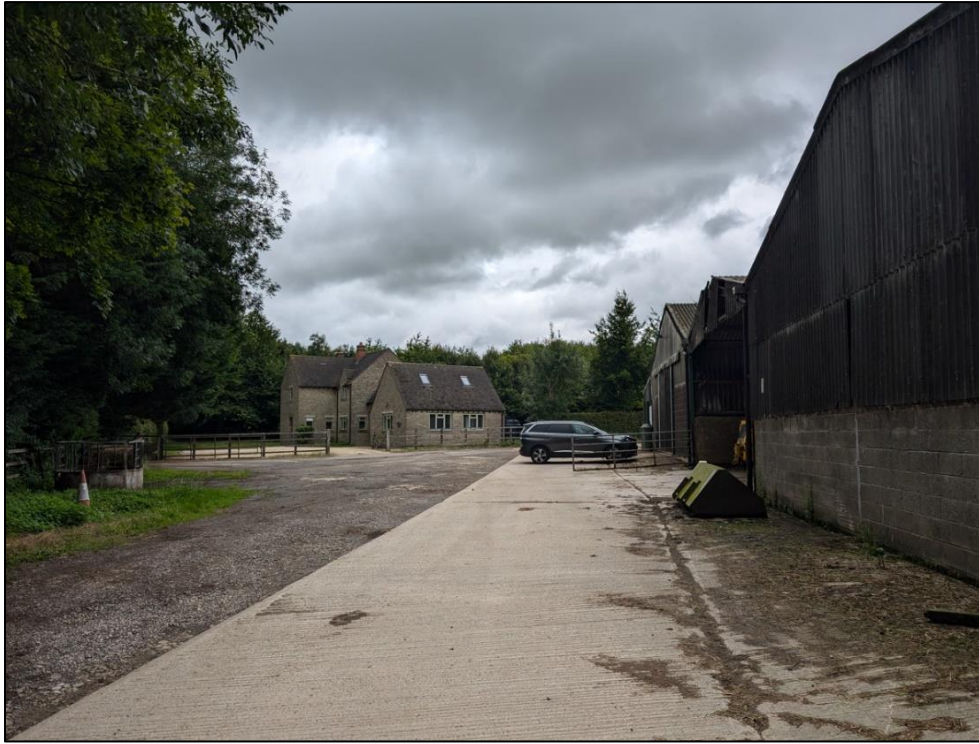
Figure 5: Existing Site Frontage and Adjacent Oakwood House
