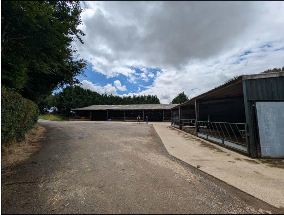
Figure 4: Existing Barn Structures on Site and Hardstanding Yard Area
