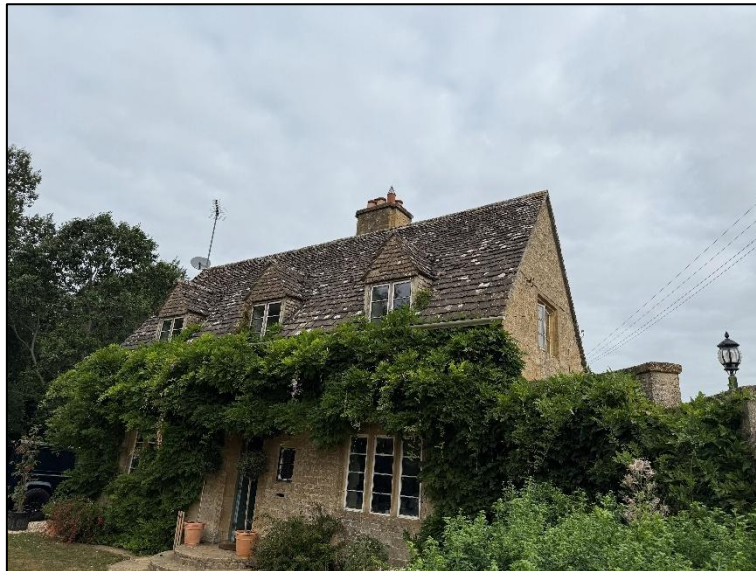
Plate 1. The front of the House as seen from the South
