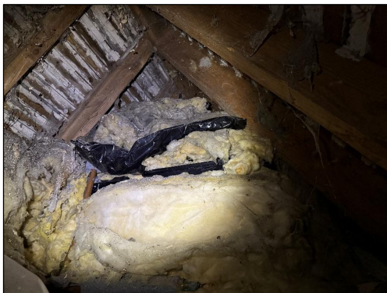
Plate 9. Insulation clutter in the Smaller of the 2 loft spaces in the House
