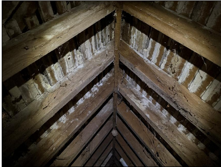
Plate 10. Image showing timber frame and torching in loft
