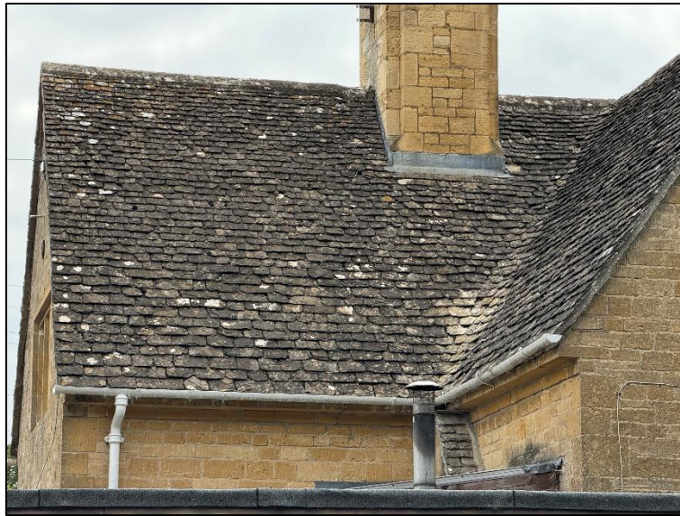
Plate 6. North-western roof sections, tiles and stone eaves
