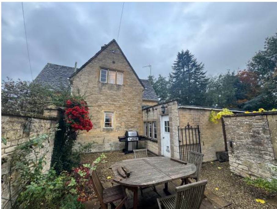
Photo 3 – existing elevation to courtyard
