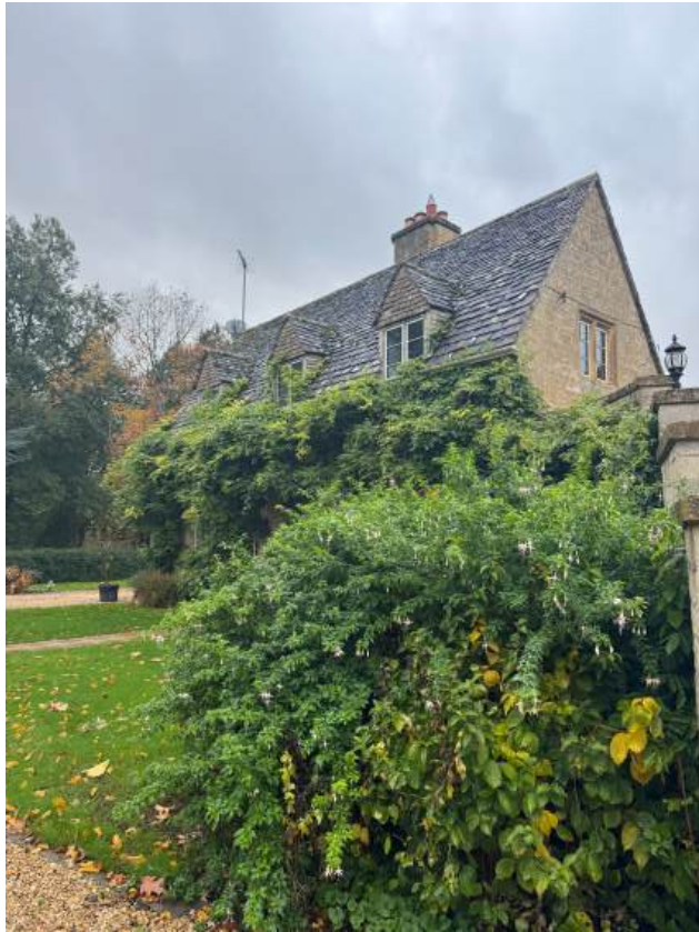
Photo 4 – front elevation viewed from the access off Small House Lane
