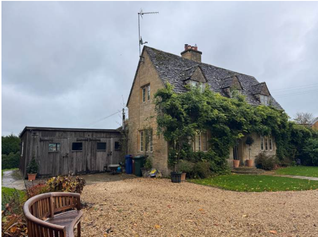
Photo 1 – existing front elevation – note the timber weatherboarding to the garage
