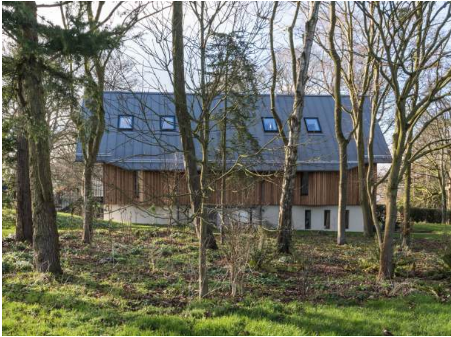
Photo 7 – east elevation of The Long House completed, facing towards The Small House – note the use of metal standing seam roofing and vertical timber weatherboarding (which has since silvered)
