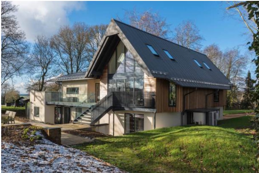
Photo 6 – south and east elevations of The Long House completed – note the use of metal standing seam roofing and vertical timber weatherboarding (which has since silvered)
