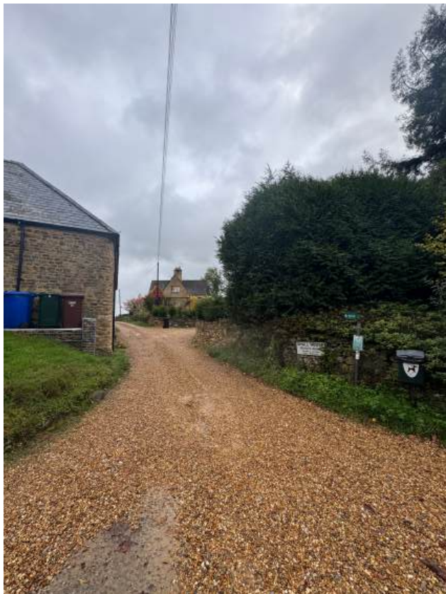
Photo 5 – north elevation viewed from the entrance to Small House Lane, off Main Street
