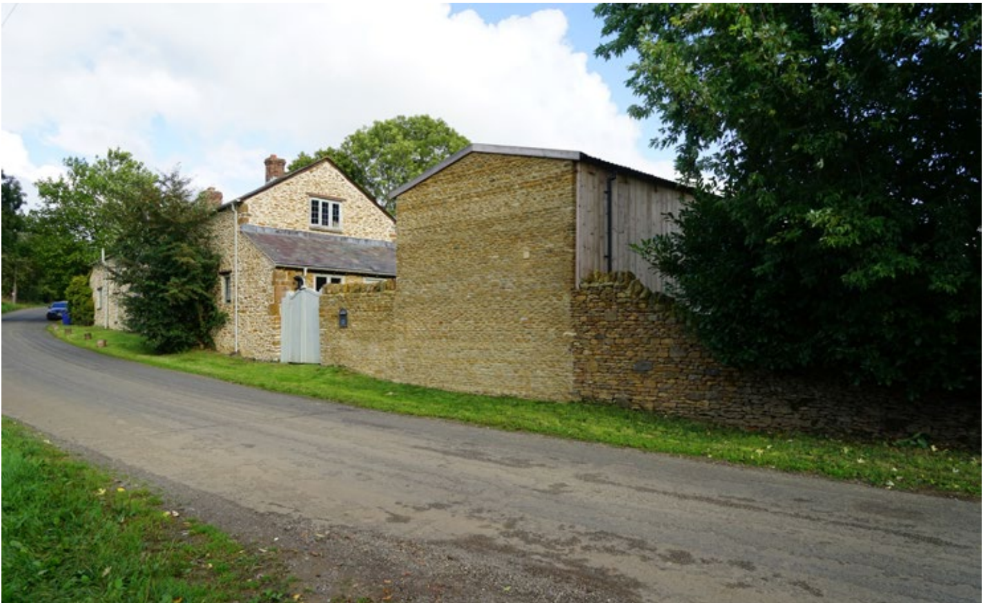
View from the north-east showing the relationship between the cottage and the new garden room, which while the height to the eaves is higher than the approved structure, is nonetheless, considered modest relative to the scale of the cottage.
