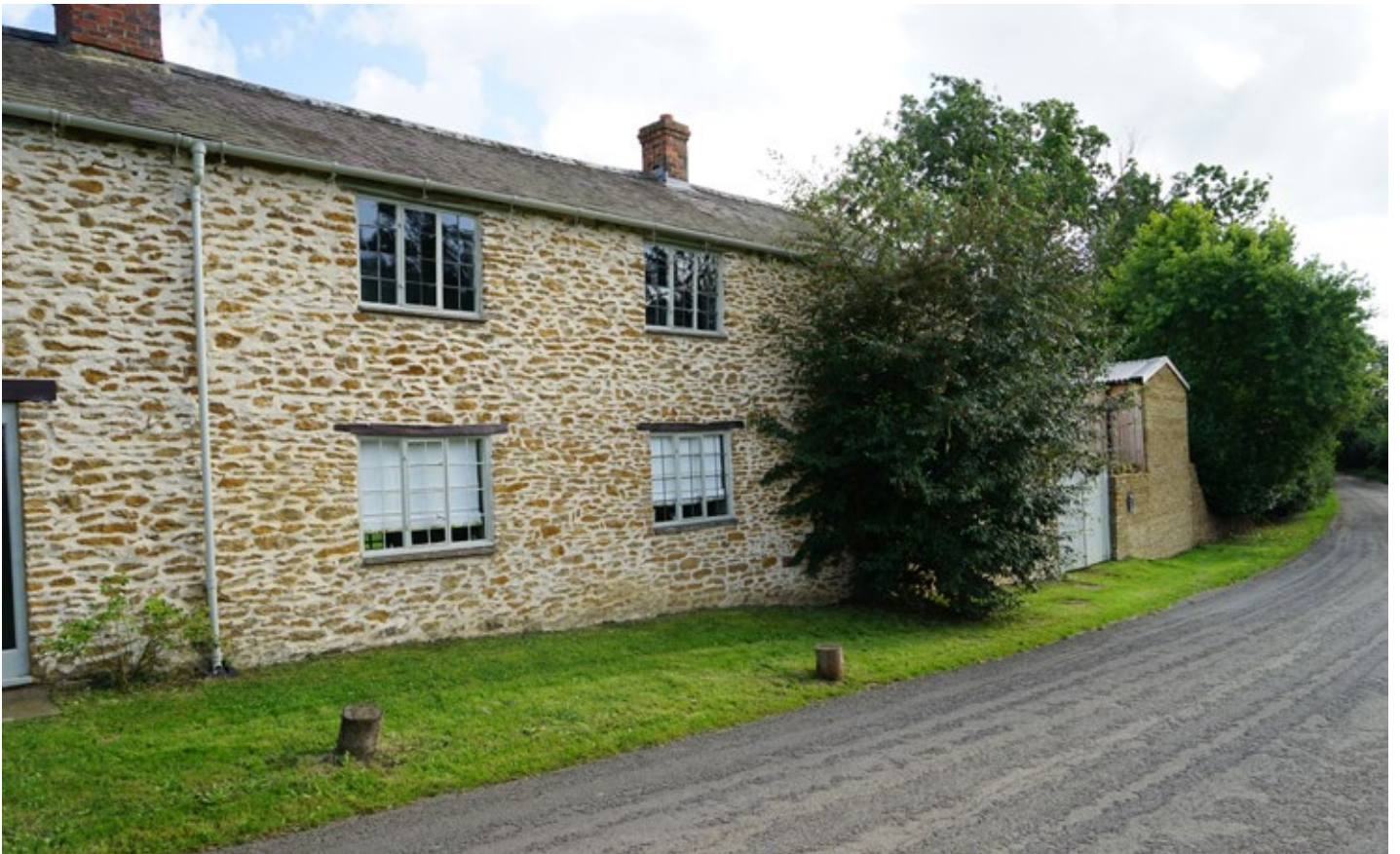
View from the north-east showing the relationship between the cottage and the new garden room, which while the height to the eaves is higher than the approved structure, is nonetheless, considered modest relative to the scale of the cottage.
