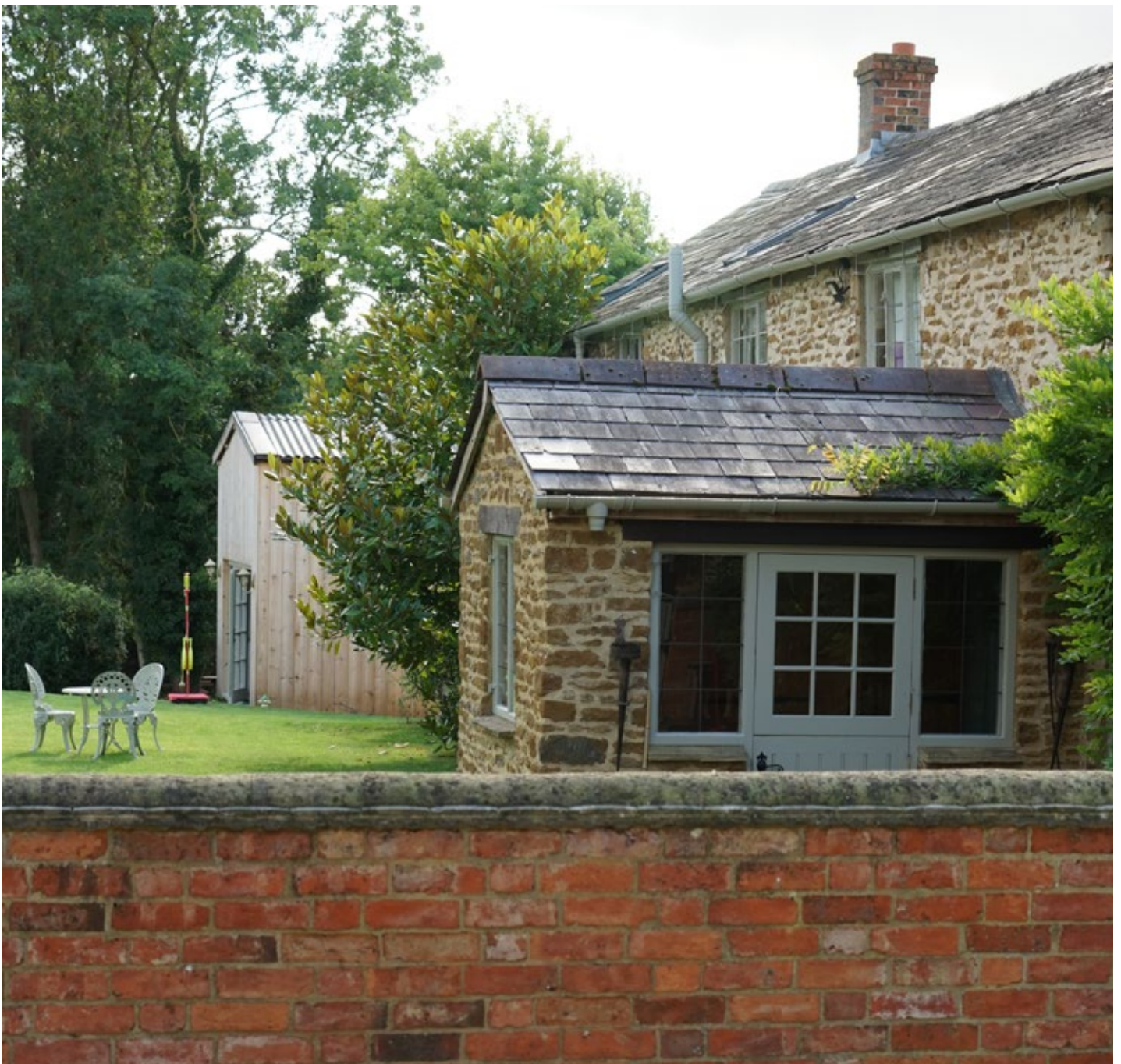
View showing the pitch of the garden room as built and of the shallow pitch of the rear porch
