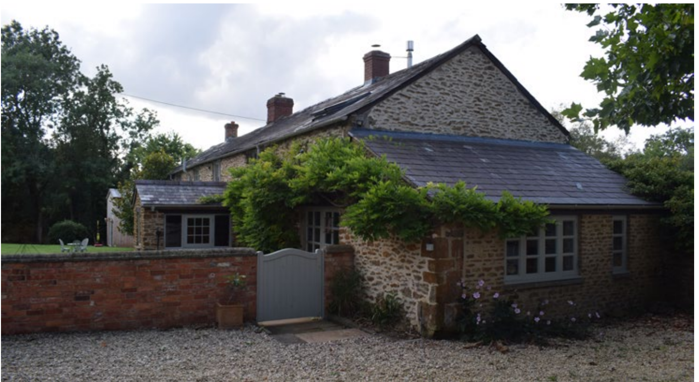
View from the north of the former cottage no. 7 with timber casement windows in contrast to No. 8 with metal casements.
