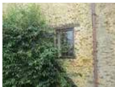
Existing North West Elevation - far right window
