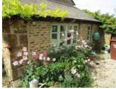
Stone wall of north west elevation - low level
