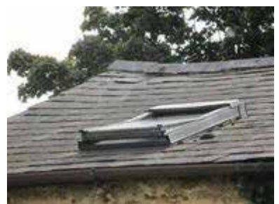
Existing North West Elevation - roof lights
