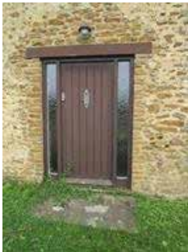
Existing main entrance door
