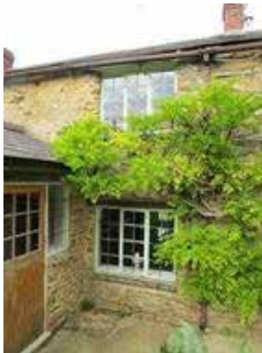
Existing South East Windows - right of porch
