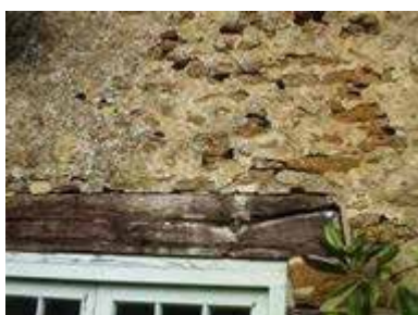
Existing timber lintel to Games Room door
