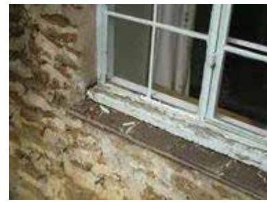
Existing South East 1st Fl Window - cill
