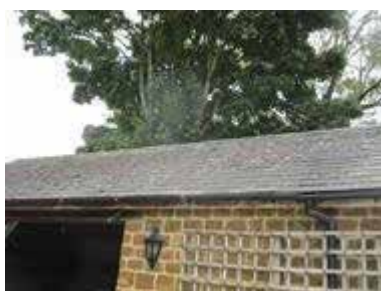
Existing slate roof tiles of garage
