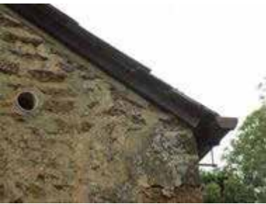
Stone wall of north east elevation - top right between rafters and sloped roof
