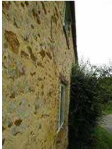
Stone wall of north west elevation - right hand side of right hand chimney stack
