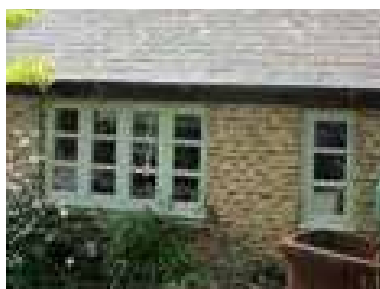
Existing North East Elevation - windows
