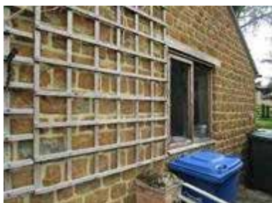
Existing south east facing window of garage
