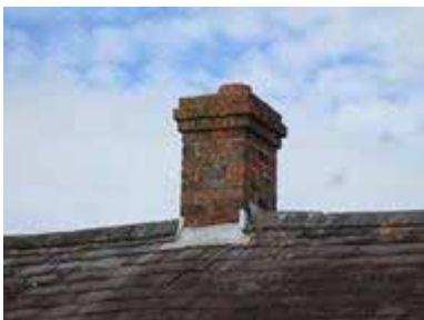
Existing Chimney Stack - Left
