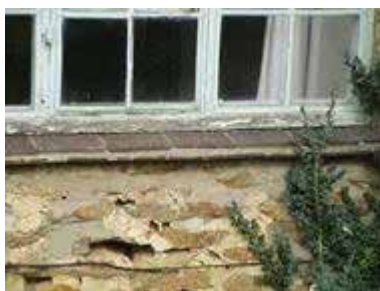
Stone wall generally between central and left hand chimney stacks
