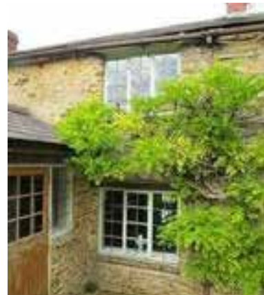
Stone wall right of entrance porch
