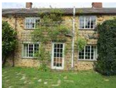
Existing South East 1st Fl Window - between central stack and left hand stack
