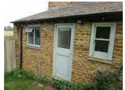
Existing South West Elevation - ground fl windows
