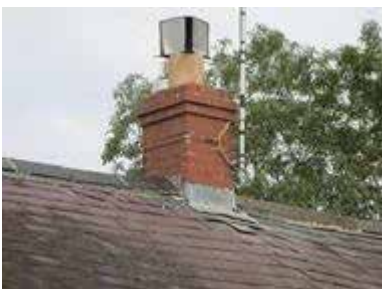
Existing Chimney Stack - Right
