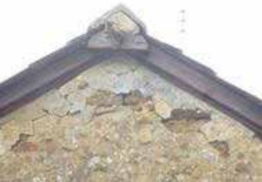
Stone wall of north east elevation - gable
