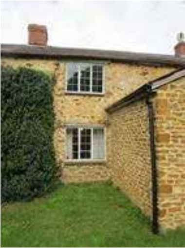
Stone wall left of entrance porch
