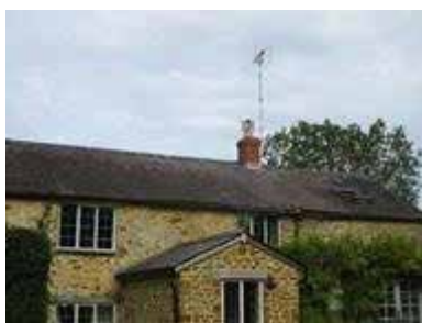
Existing South East Roof lights - right side
