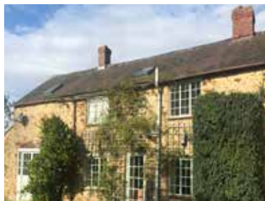
Existing roof ridge - left side
