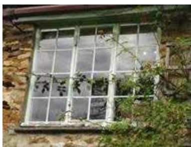
Existing South East Windows - Crittall style
