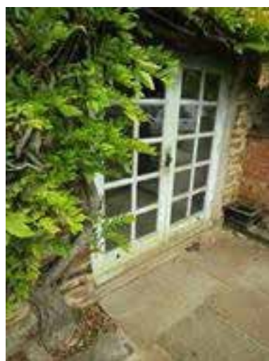
Existing double doors to right of this elevation
