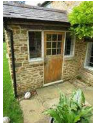
Existing South East Windows - right of porch
