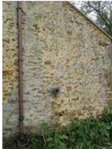
Stone wall of north west elevation - far right - wall to "garden room"
