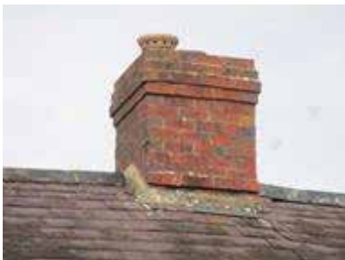
Existing Chimney Stack - Central
