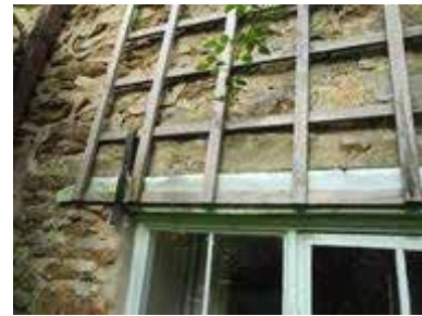
Existing South East 1st Fl Window - lintel
