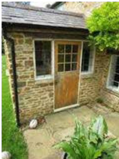
Existing “stable” style side entrance door
