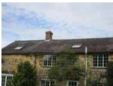
Existing South East Roof lights - left side
