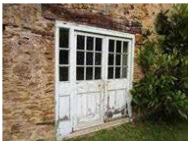
Existing door to Games Room
