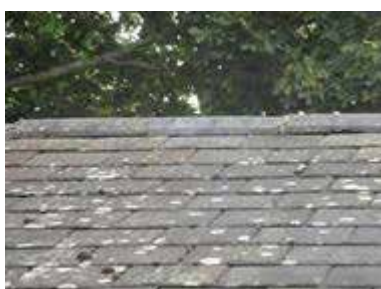
Existing slate roof tiles of garage
