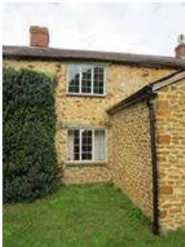
Existing South East Windows - left of porch
