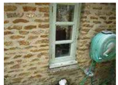
Existing North East Elevation - window left
