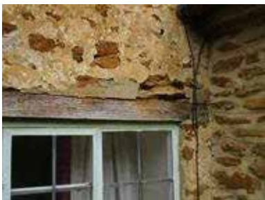
Existing South East Windows - right of porch
