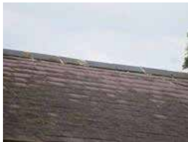
Existing roof ridge
