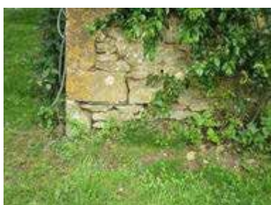
Stone wall outside of small single storey extension to the far left of property
