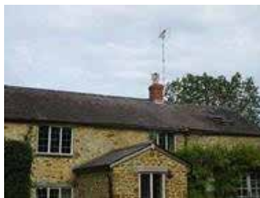
Existing roof ridge - right side
