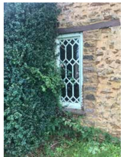
Existing North West Elevation - window with honeycomb glazing
