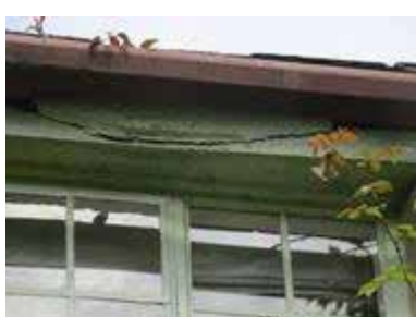
Existing North West Elevation - 1st Fl Windows - lintels
