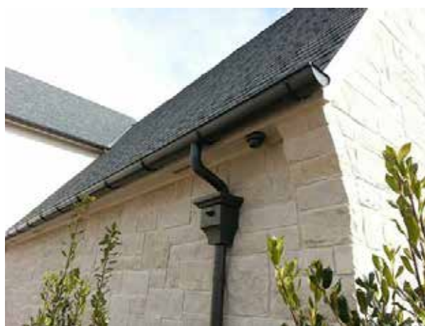
Similar conservation painted metal gutter and down pipe system
