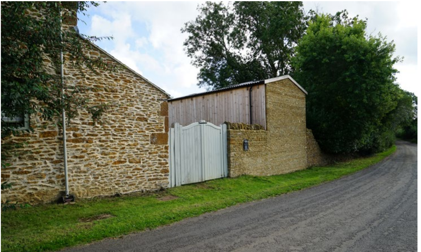
View showing relationship and scale between the lean-to portion of the cottage and the new garden room which is located on the historic site of the 1845-51 barn. The use of stone for the north gable – the original barn was stone, visually ties the building to the boundary walls and cottage
