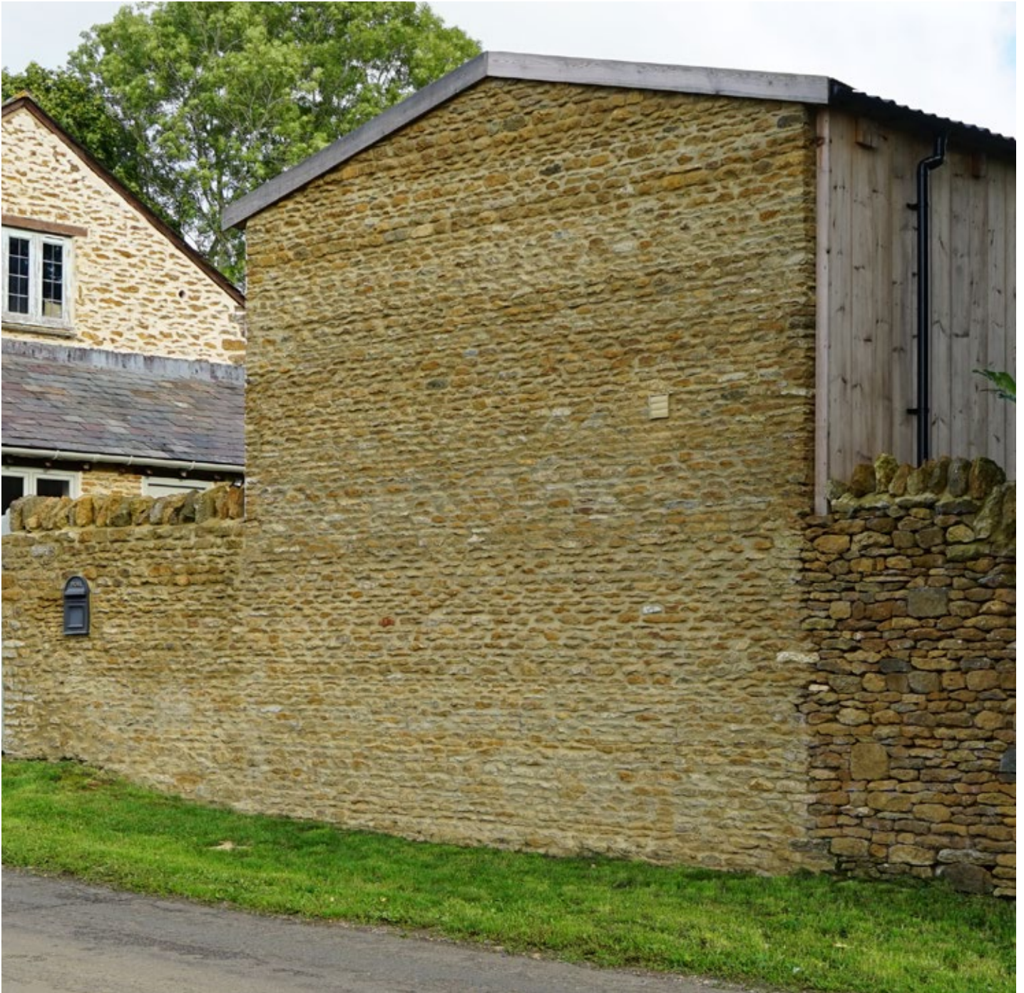
Image of the new garden room from the north, with stone to the roadside and vertical timbers to the sides
