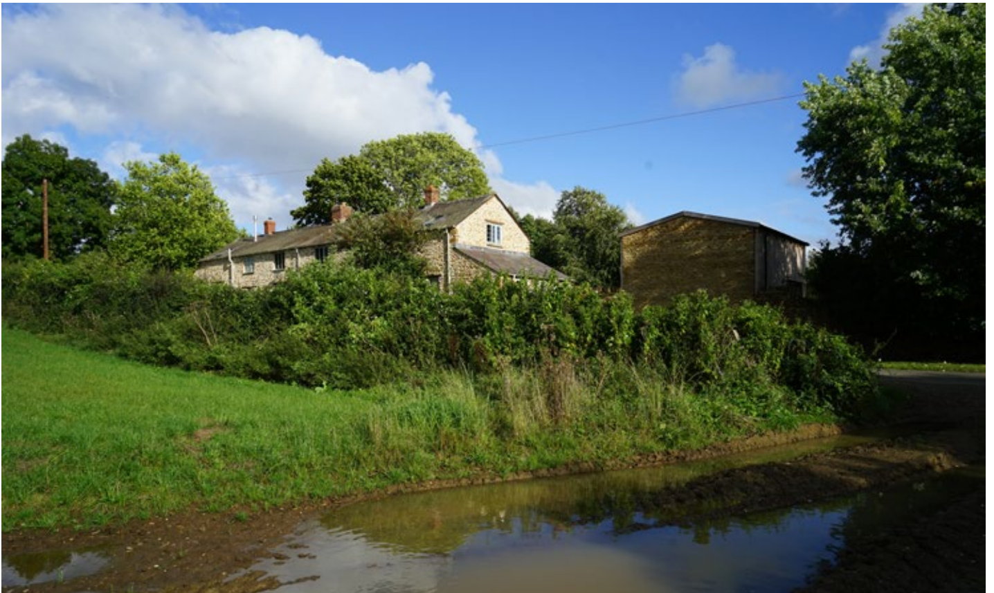
View from lane to the north looking back towards Bartlett Cottage. There is a clear visual separation between the garden room, which has been constructed to the approved ridge height, but with increase high to the eaves. It is not considered the garden room as built, as a contemporary structure, detracts from the visual appreciation of the cottage and its rural and garden setting.
