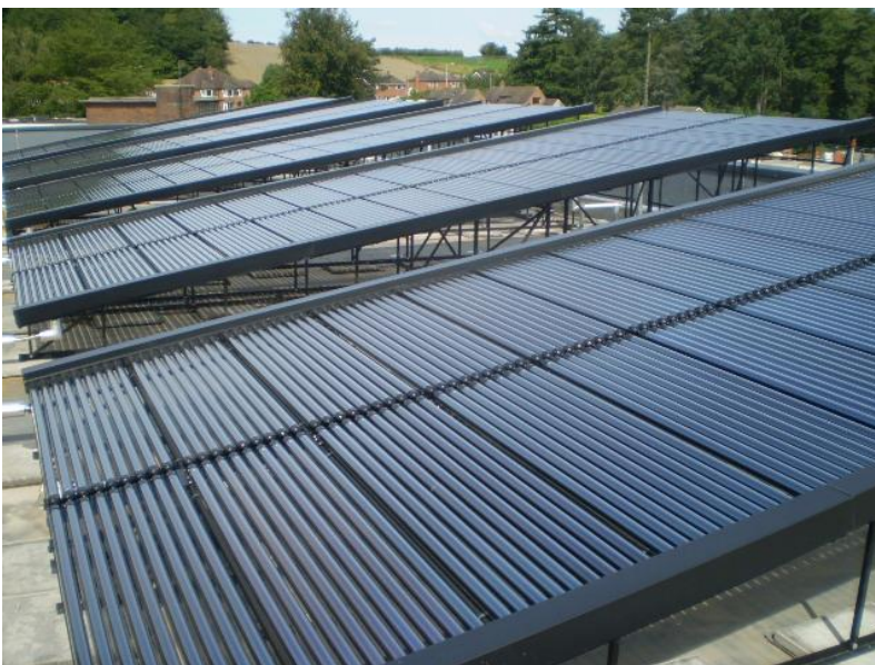
Figure 5 - CPW Solar Thermal Evacuated Tube Systems: William Brookes School (left) and Police Federation Headquarters (right)
