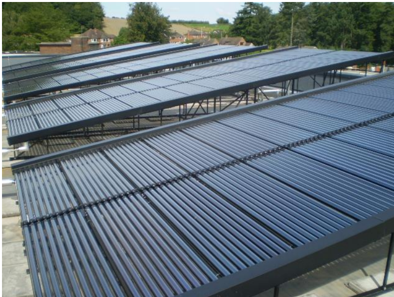
Figure 5 - CPW Solar Thermal Evacuated Tube Systems: William Brookes School (left) and Police Federation Headquarters (right)
