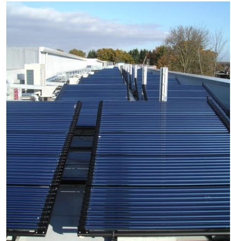
Figure 5 - CPW Solar Thermal Evacuated Tube Systems: William Brookes School (left) and Police Federation Headquarters (right)
