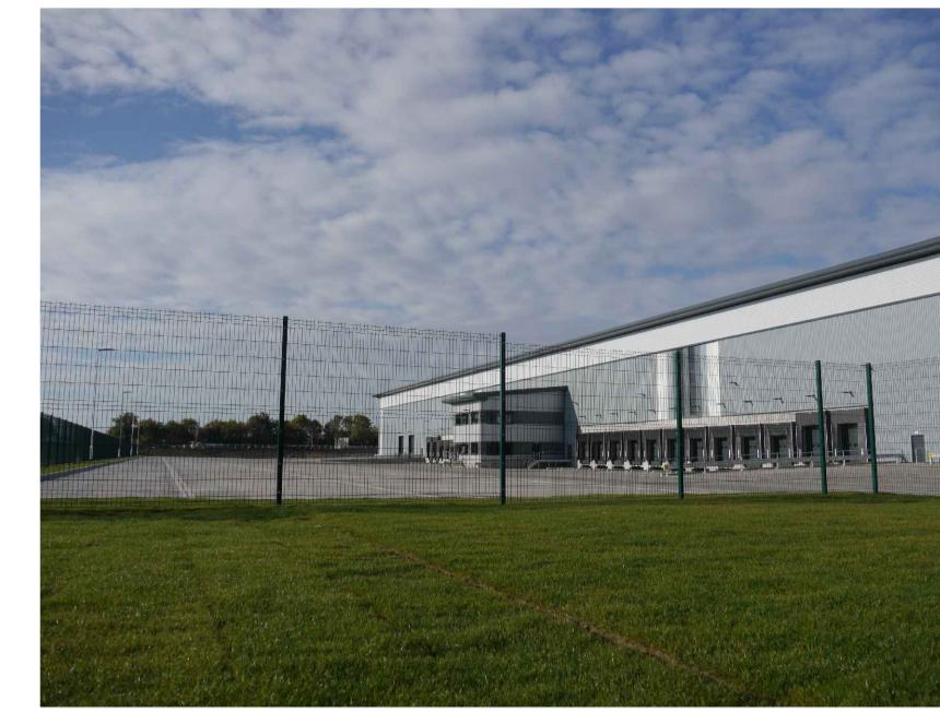
Image of typical paladin mesh security fence
