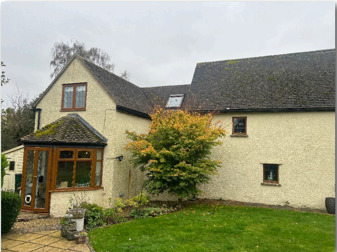
The above photo shows the “rear” (North elevation) of the existing cottage looking towards the bay window that is proposed to be demolished and replaced with a garden room extension.
