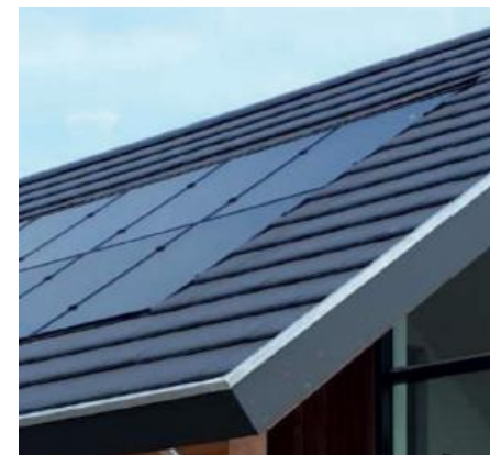
In roof solar panels
