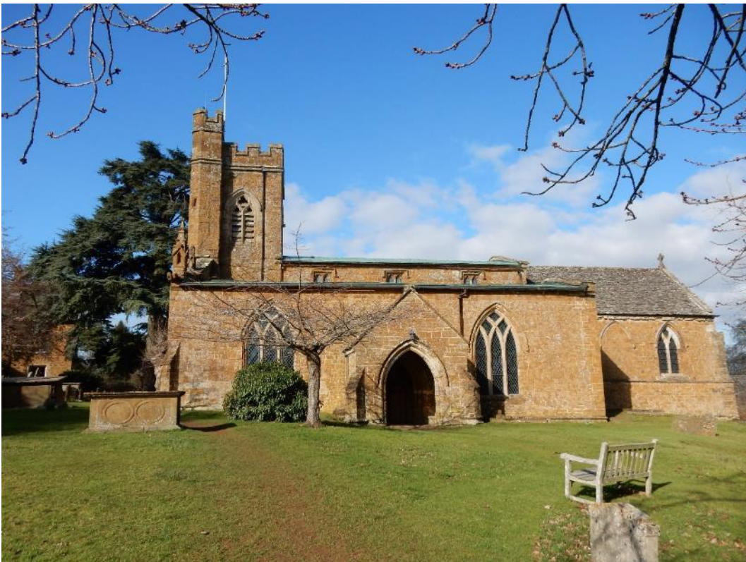
Plate 14: South elevation of St Peter's Church, from churchyard
