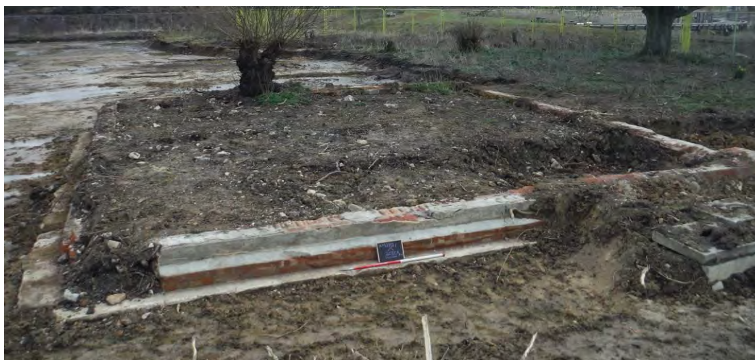
Plate 5: Building footprint 2038, and concrete foundation 2037
