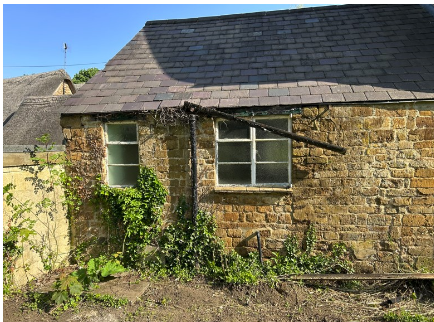
Fig.1 & 2 – existing single storey side addition
