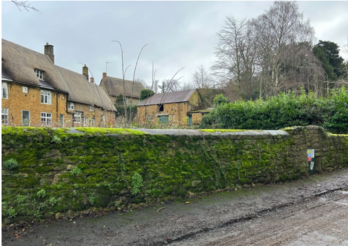
Fig.9 – Church Street – existing boundary wall
