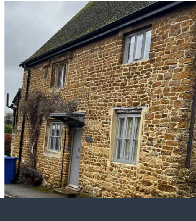
Local Ironstone and timber window heads
