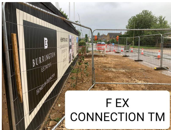
S106 Foul Connection location on Hempton Road
