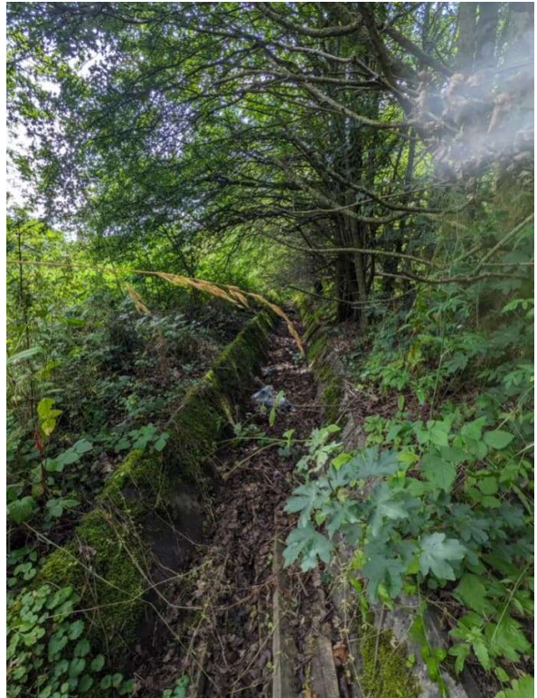
Figure A.12: Existing ditch east of southern site
