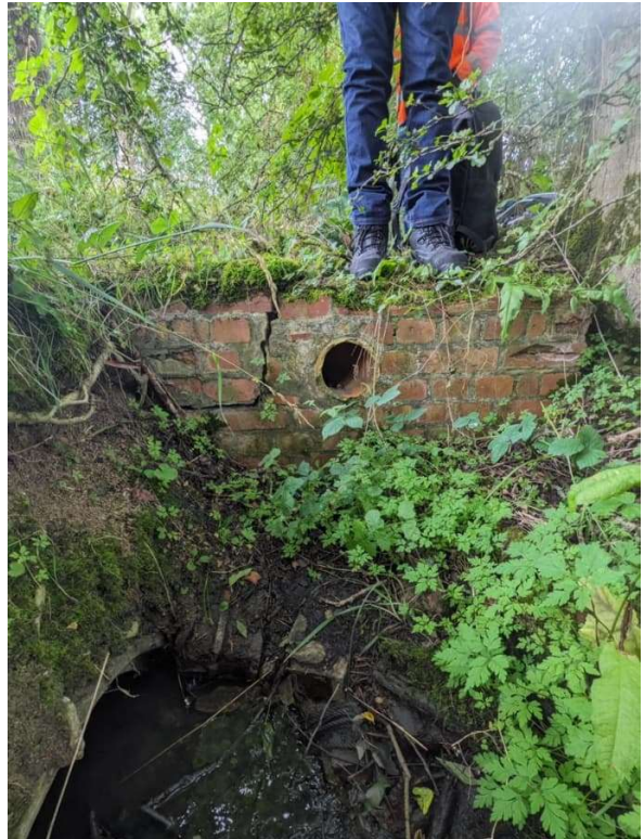
Figure A.10: Outlet within wall adjacent culvert
