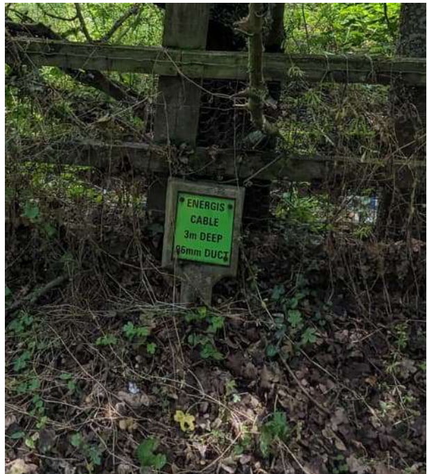
Figure A.16: Existing utility marker post located in southeast corner of site
