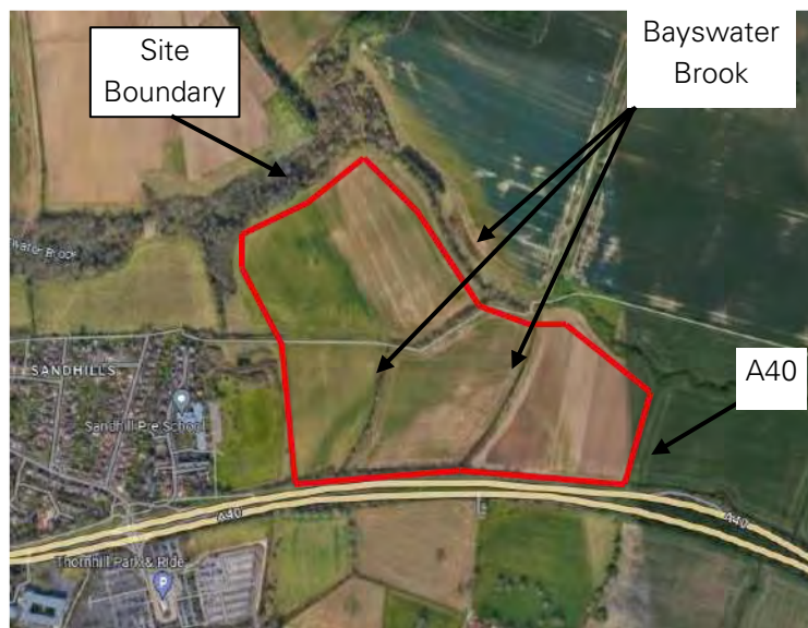
Figure 3a: Aerial view of Land North of Thornhill Park and Ride with Approximate Site Boundary (Google Maps, 2023)
