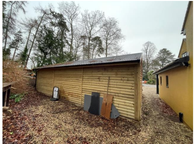
Photograph 10. The garage viewed from the west.
