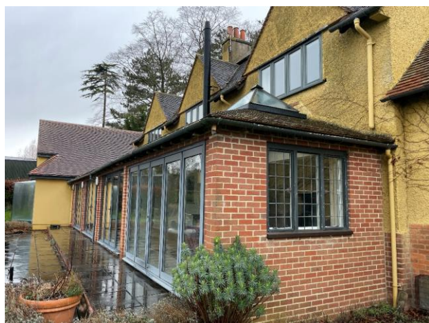
Photograph 6. The dwelling (showing the rear modern extension) viewed from the south-east.
