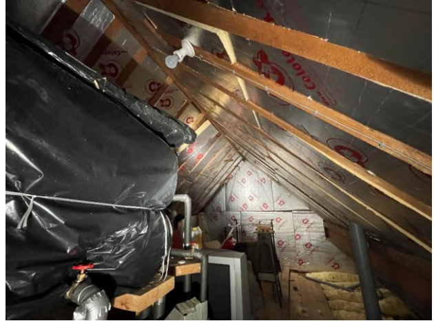
Photograph 8. The loft space above the three-storey section of the dwelling.
