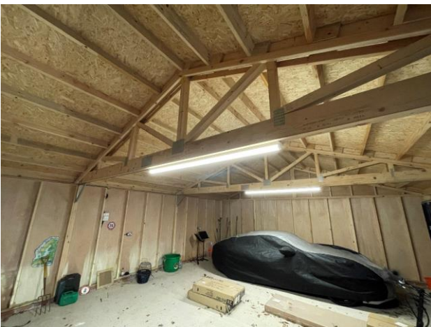
Photograph 11. The interior of the garage.
