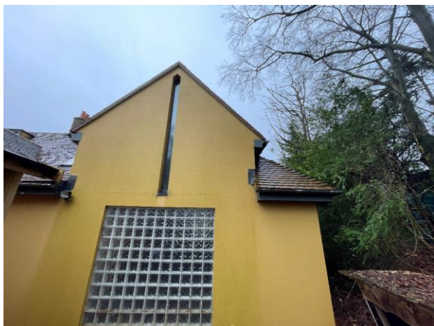
Photograph 3. The dwelling (showing the swimming pool wing) viewed from the north.
