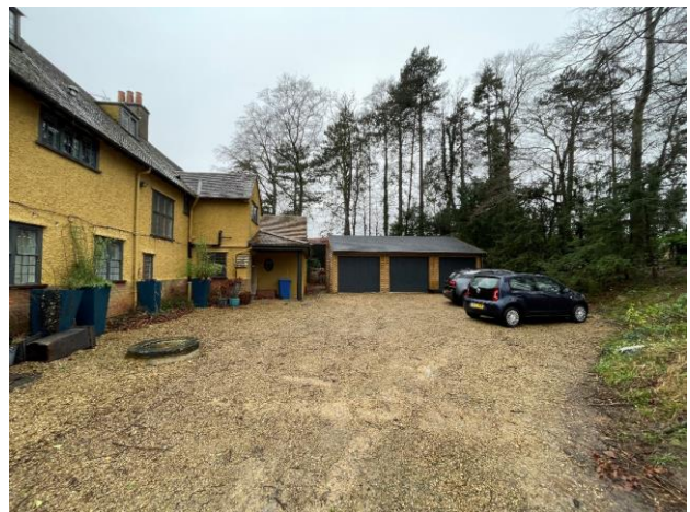
Photograph 12. The gravel hardstanding surrounding the dwelling and garage.
