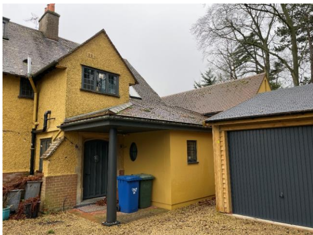
Photograph 1. The dwelling (showing the front gable) viewed from the north.
