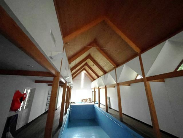
Photograph 7. The interior of the swimming pool wing.
