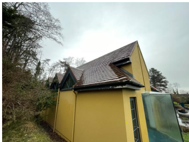
Photograph 4. The dwelling (showing the swimming pool wing) viewed from the south-west.
