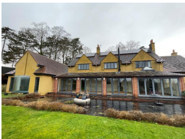
Photograph 5. The dwelling viewed from the south.
