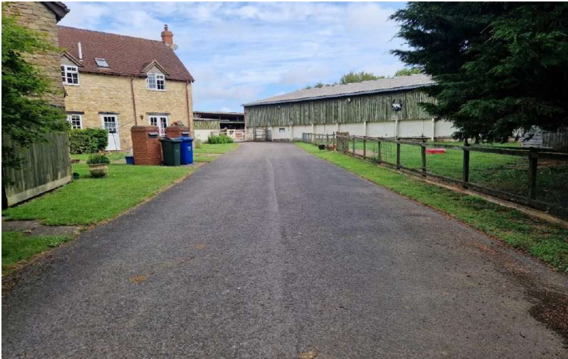
Image EDP A1.9: Tarmacked access track through the Site.
