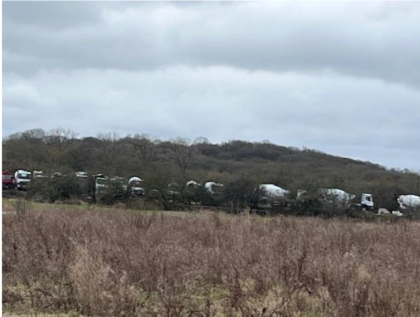
Fig. 5 Ready-made concrete lorries viewed across site from entrance on Widnell Lane
