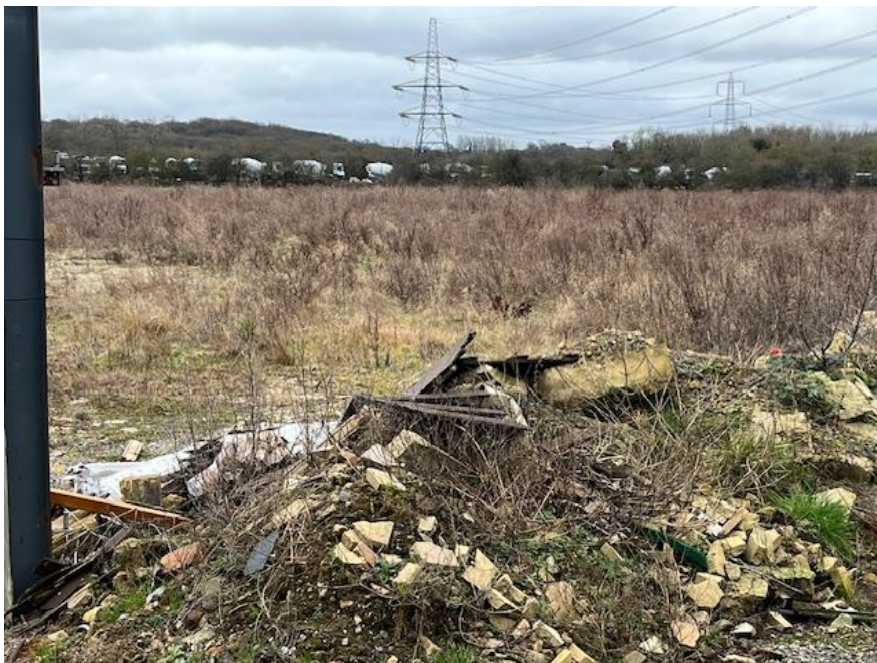
Fig. 2 The site entrance (with a view of ready-made concrete lorries beyond)
