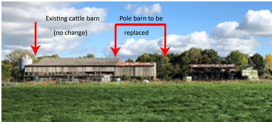
West elevation, illustrating the existing barn and the pole barn addition to be replaced by the Proposed Extension
