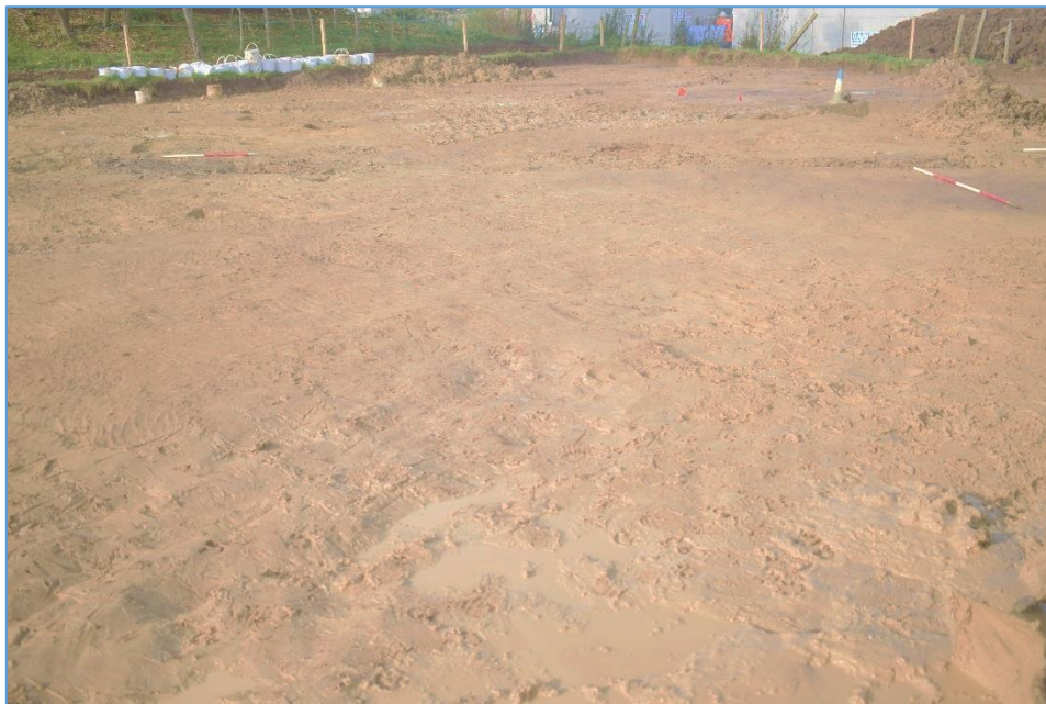
Plate 35: Working shot of North Area, looking west
