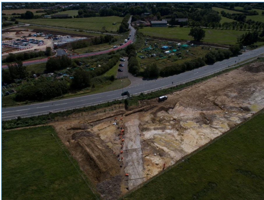
Plate 30: Drone imagery of road D(3311), looking south-east
