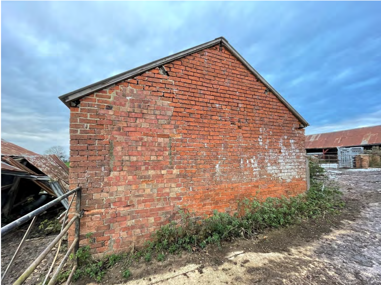
Plate 17: West range, south flank elevation.
