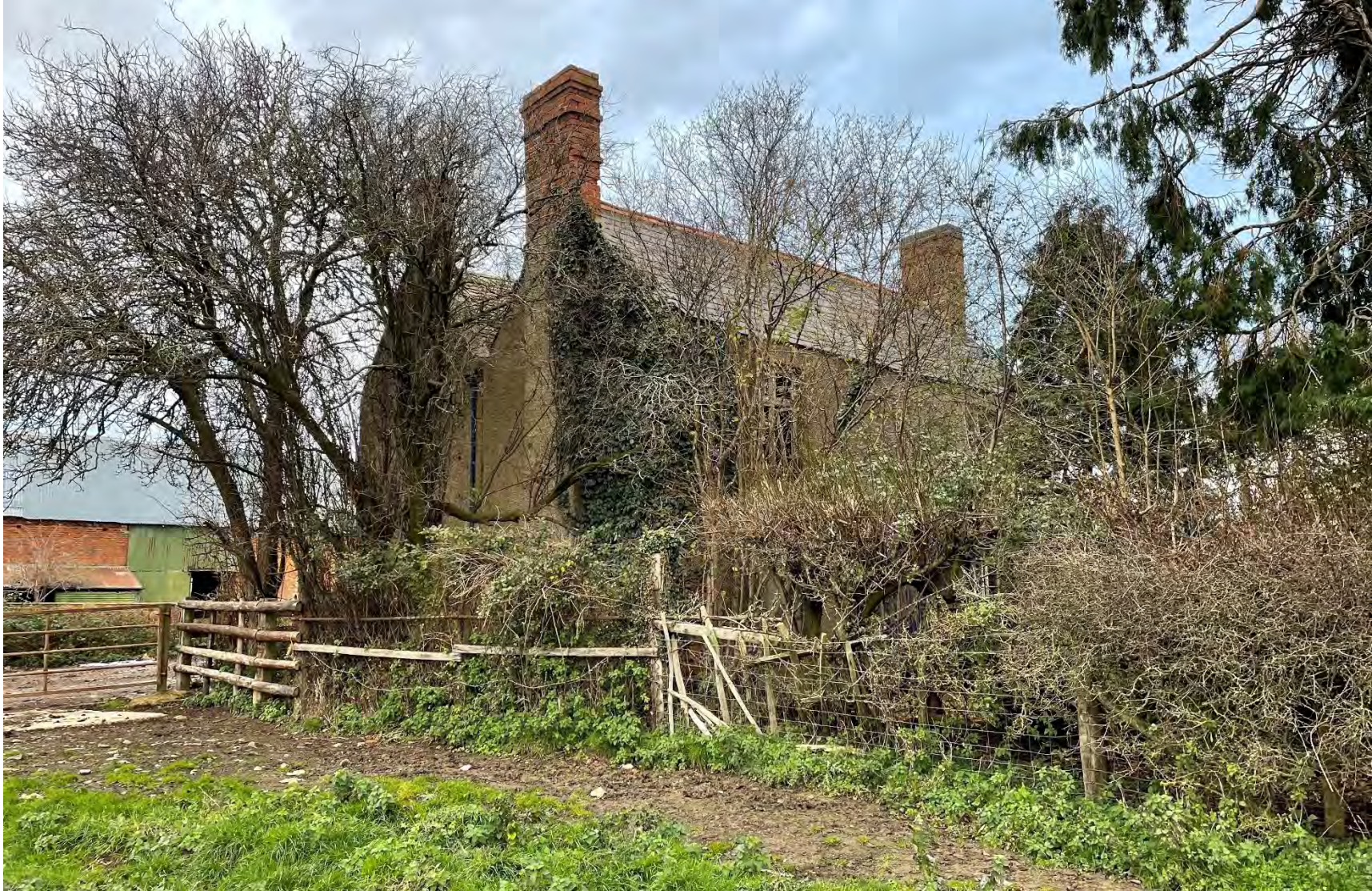
Plate 14: Huscote Farmhouse, west flank and rear elevations.
