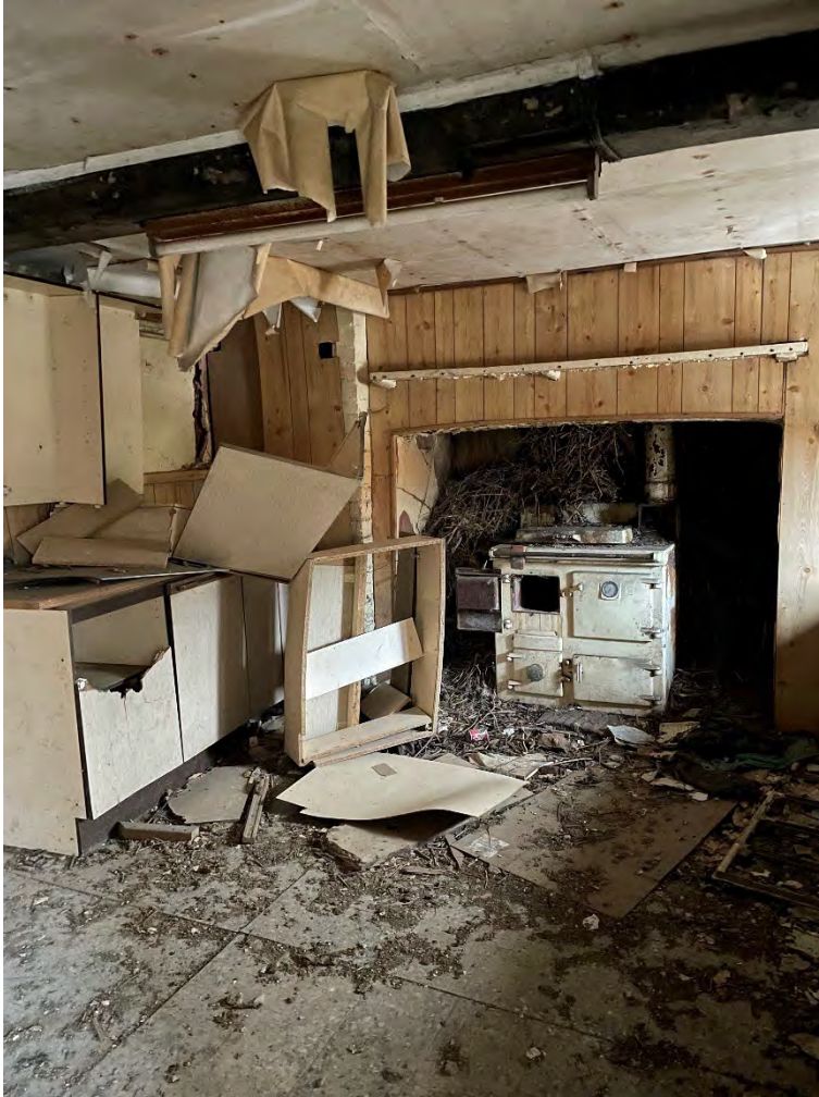
Plate 15: Huscote Farmhouse, interior of kitchen.
