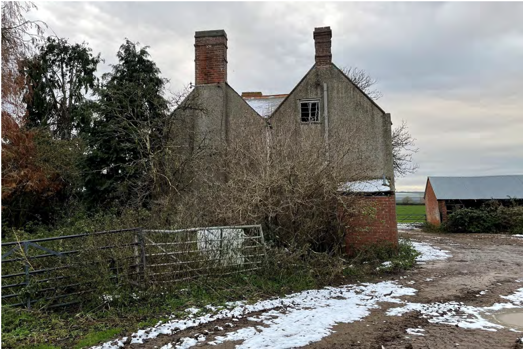
Plate 13: Huscote Farmhouse, east flank elevation.
