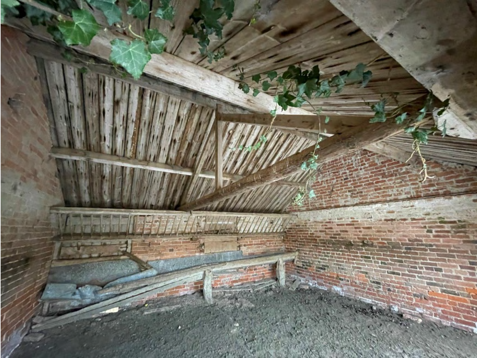
Plate 18: West range, detail of interior.
