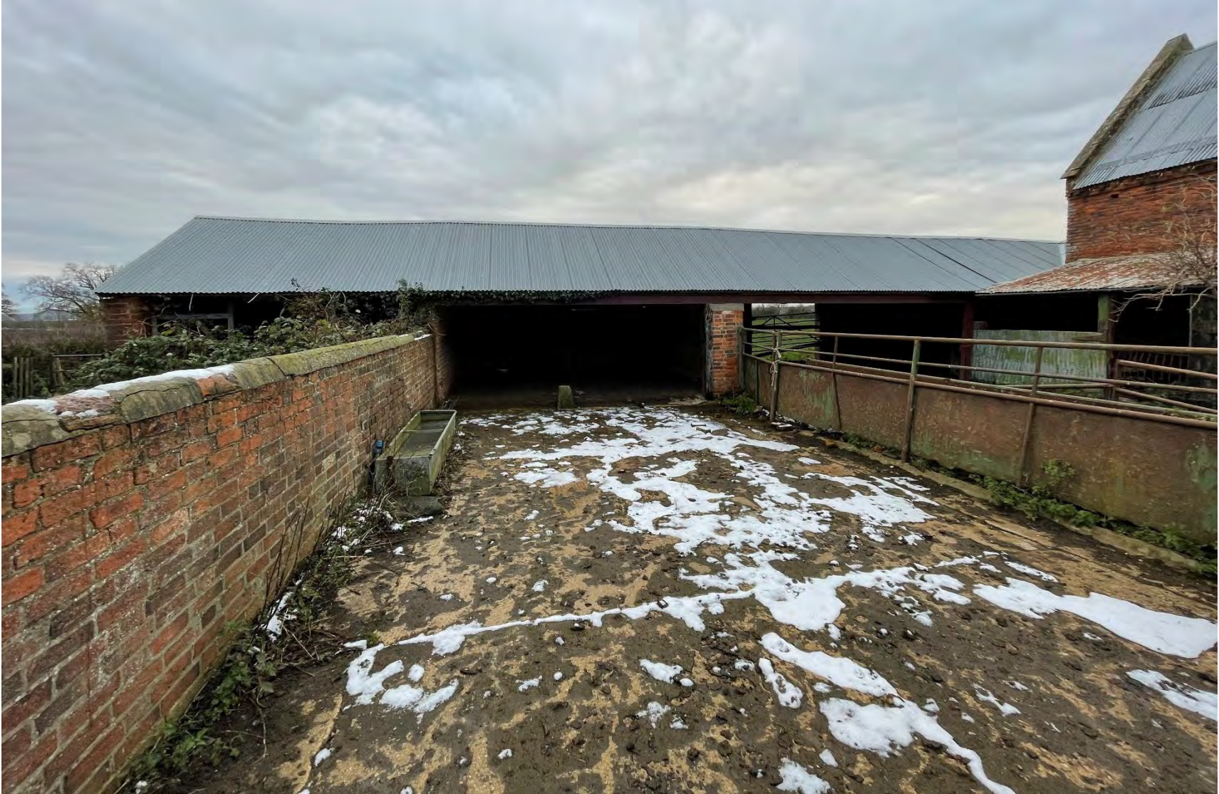
Plate 16: West range, east elevation.
