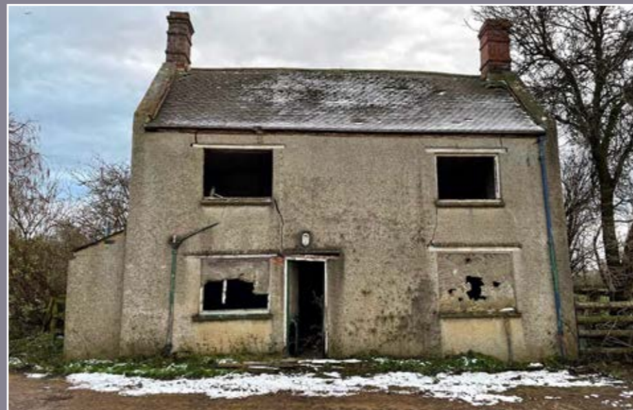
HUSCOTE FARMHOUSE, NORTH ELEVATION
