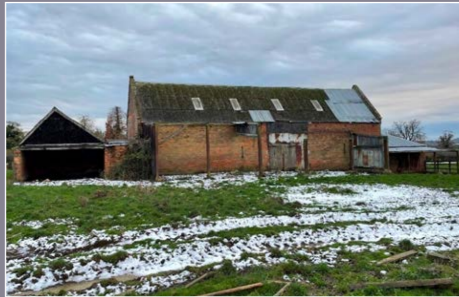
NORTH RANGE, NORTH ELEVATION
