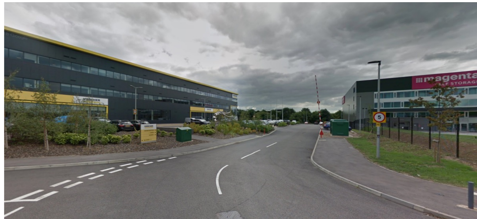
EXISTING EMPLOYMENT WEST OF THE M40 (SOURCE: GOOGLE MAPS)
