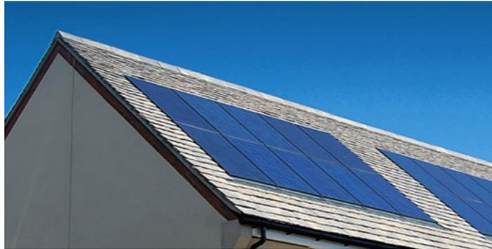
*Figure 9: Typical PV installation to pitched roof.*
