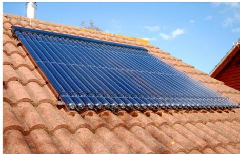
Figure 6: Typical solar thermal panel
