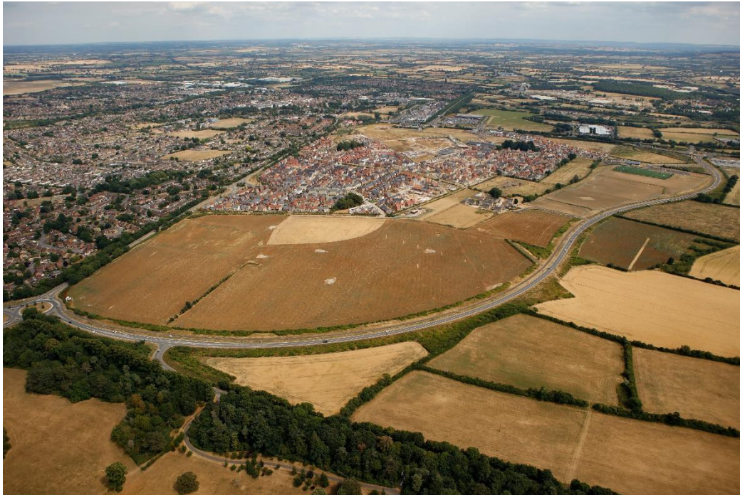
Photo 1. Aerial Photograph from September 2018, showing the Site pre-clearance, with Parcel R directly in the centre of the frame.
