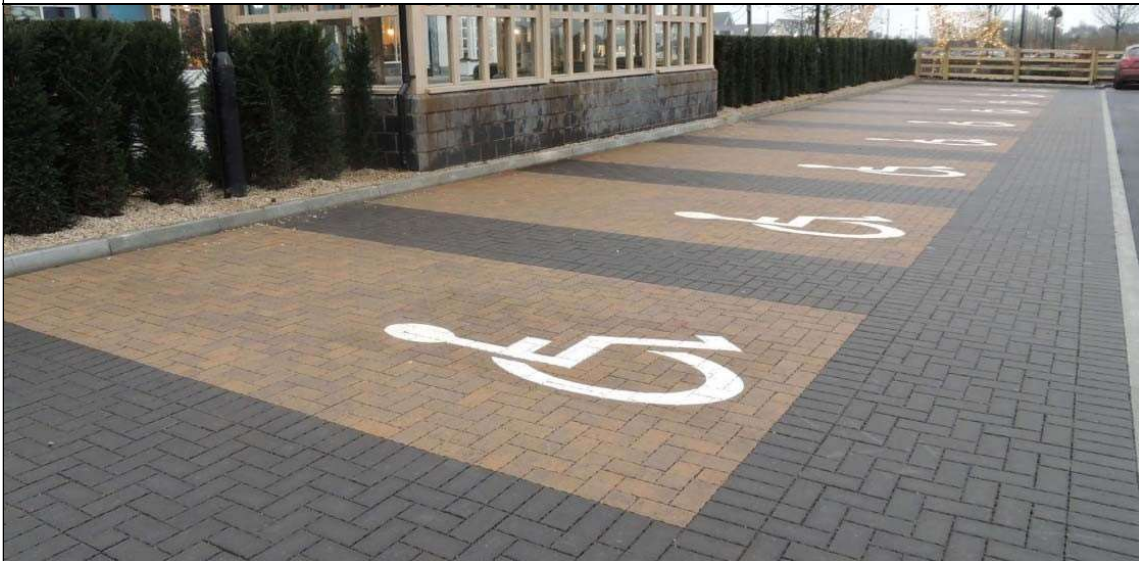
Figure 6.8: Example Block Permeable Paving
