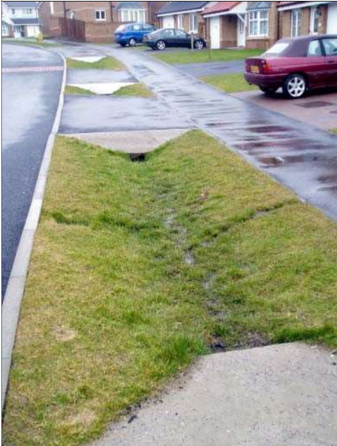
Figure 6.11: Example of Grassed Swales
