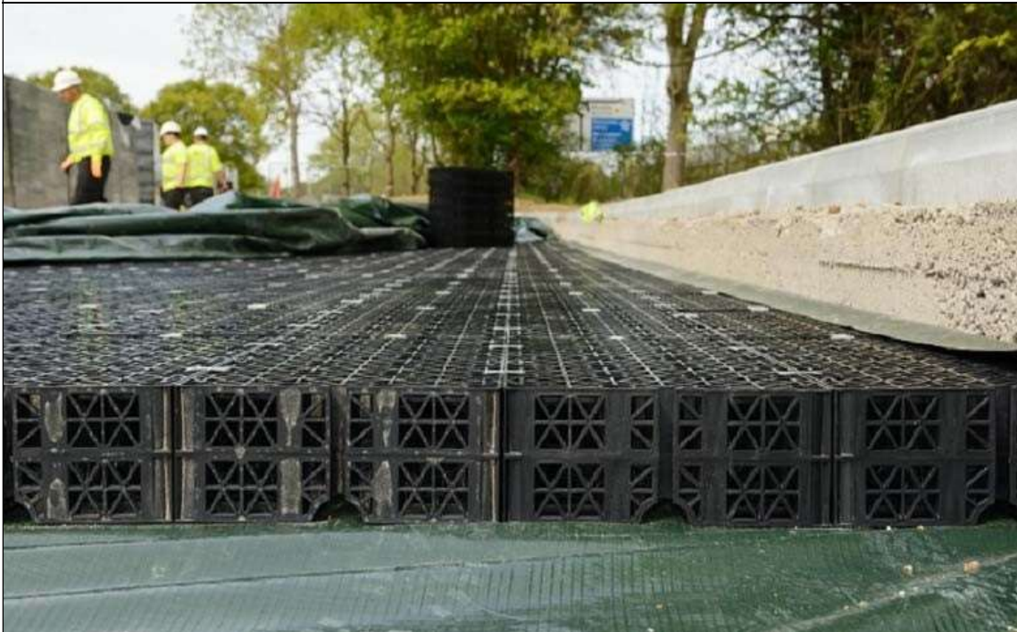
Figure 6.9: Example Crate type Attenuation Storage
