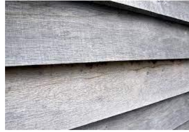
Figure 4. Self coloured horizontal oak boarding – example shows the silvering after 24months.
