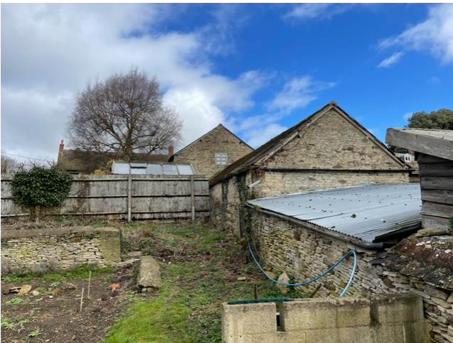
15 Defective Roofs Over Outbuildings
