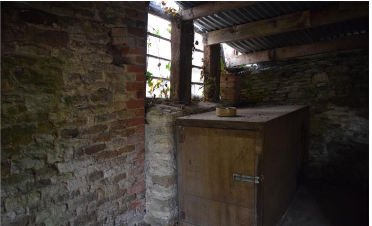
Inside the workshop showing the rear wall of the greenhouse, timber posts supporting the corrugated metal roof of the workshop and the wall to the garden beyond. Access formed into the western end of the green house and shed to form a second shower and change room
