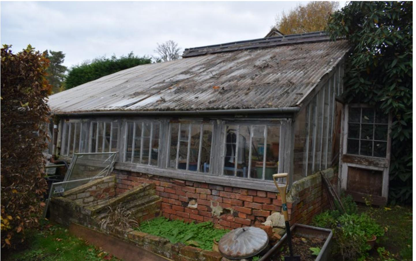
View of the lean-to greenhouse with stone and brick supporting wall to the rear. Brick base, timber windows, polycarbonate roof. Possible post WWII adaptation or rebuilding of an earlier range shown on 1919 map
