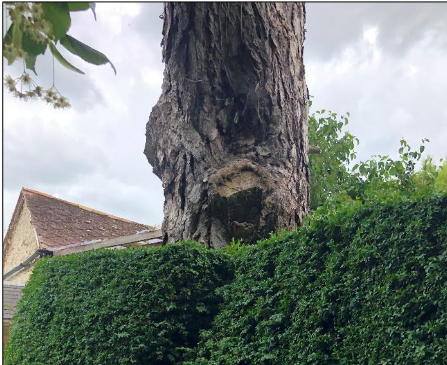
Figure 19: Rot hole at T1's south facing elevation
