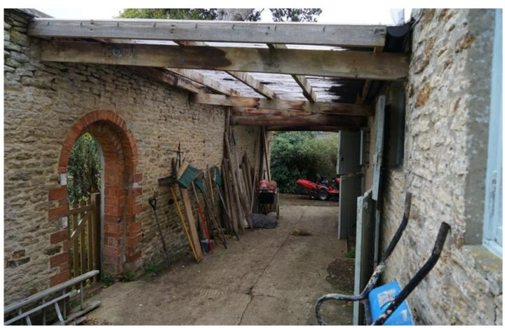
View looking south of the post 1954 stable range with later polycarbonate roof. Last stall proposed to be adapted to a plant room and shower change room
