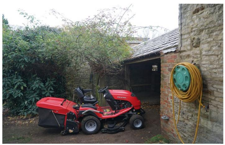
View of the end wall of the post 1954 stables, with brick pier and an infill roof spanning to the rear wall with tile capping of the greenhouse, added post 1973 map, creating a covered workshop. Slate to the yard and corrugated metal sheeting the garden side. Proposal is to replace with new glazed structure to provide garden lounge and entrance to the approved pool
