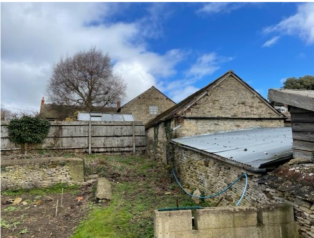
15 Defective Roofs Over Outbuildings
