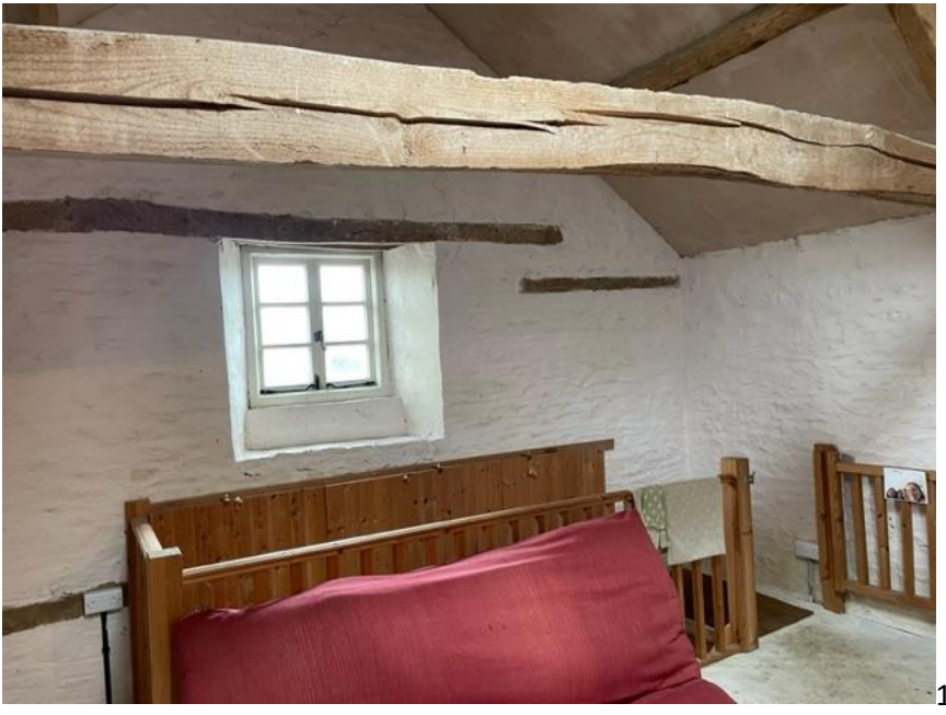
12 Upper floor of West Outbuildings
