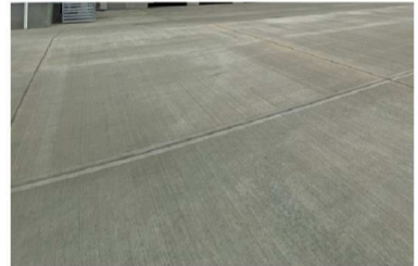
Concrete surface to concrete yard
