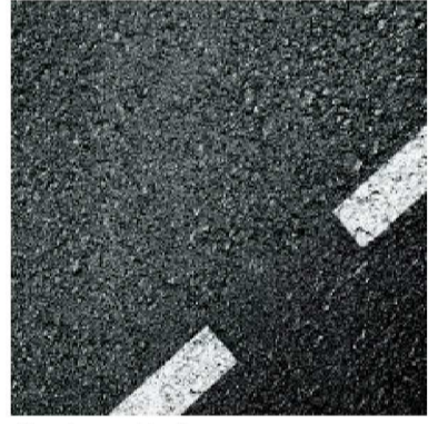
Macadam parking bays
