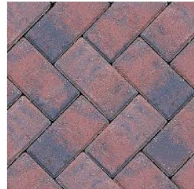
Brindle colour block paving to car park circulation aisles. Permeable paving as part of the SuDS strategy in accordance with engineers drawing : Proposed Drainage Layout T/20/2407 55-01
