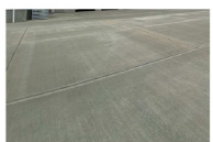
Concrete surface to concrete yard
