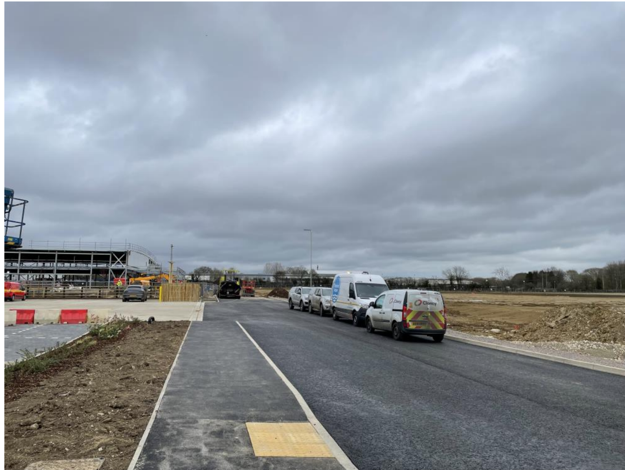
Fig. 05 Looking North Along the Internal Access Road
