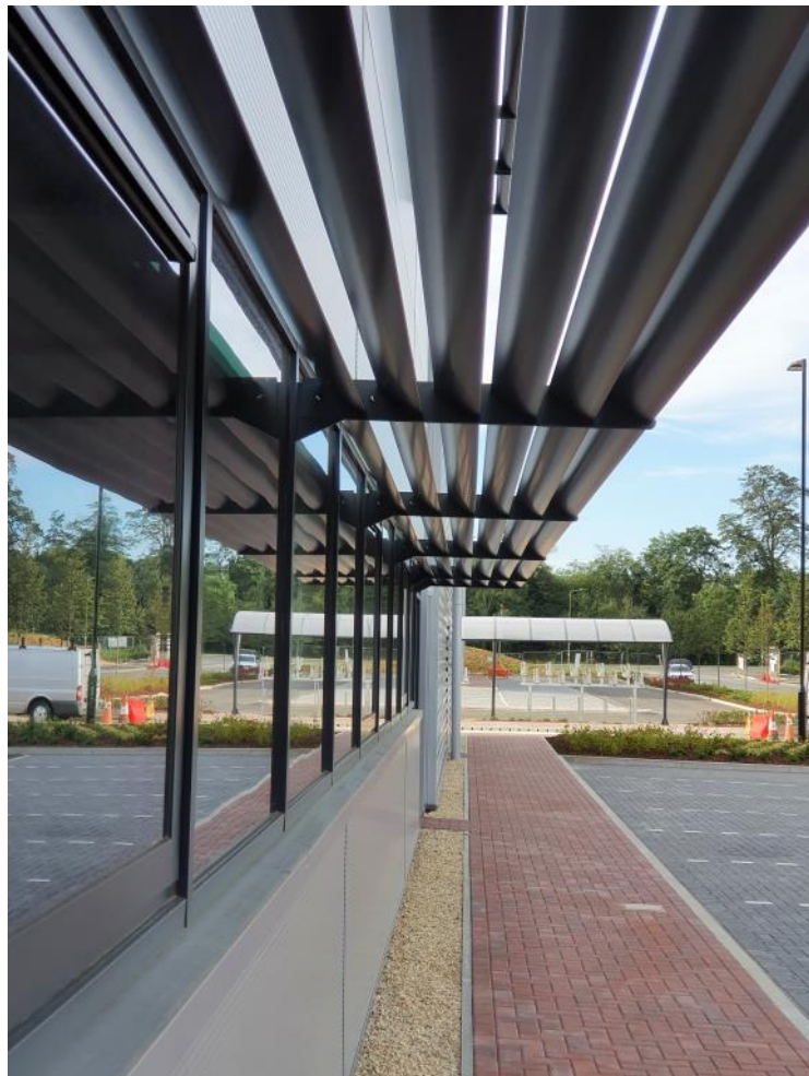
PPC aluminum glazing & brise soleil
