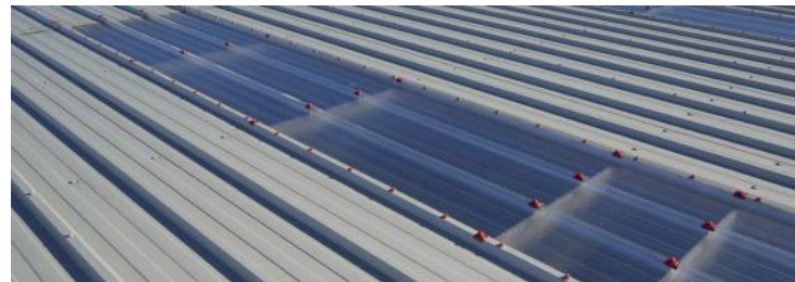
Metal profile roof & rooflight
