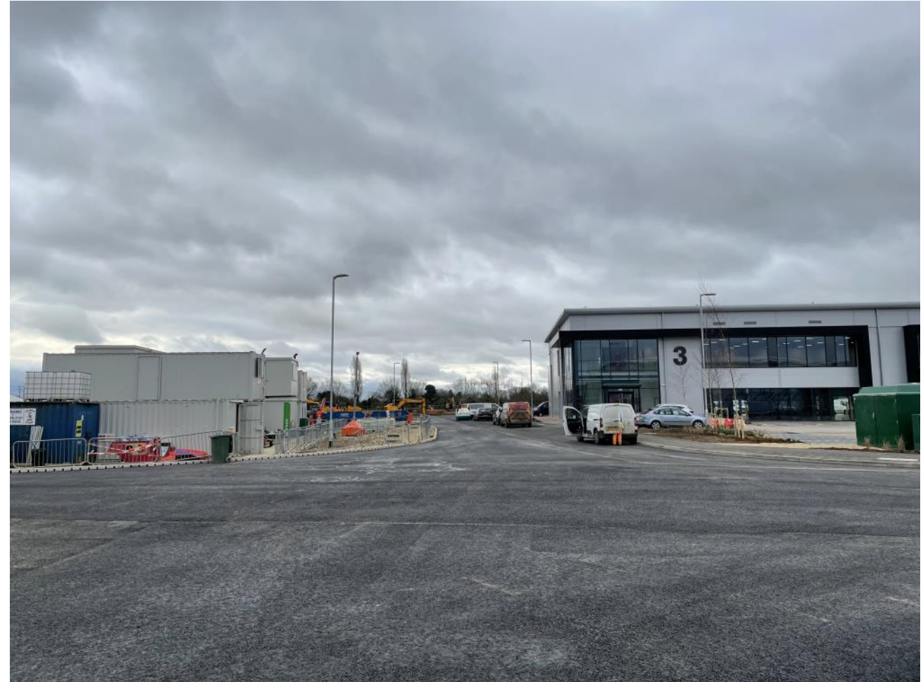
Fig. 06 Looking South Along the Internal Access Road
