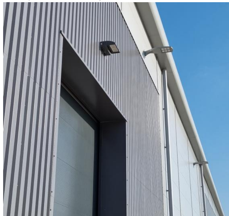
Vertical metal profile cladding & loading door
