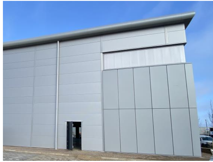
PPC aluminum rainscreen & translucent cladding
