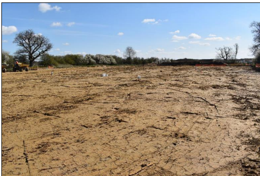
Plate 1: General view of the Site, looking northeast
