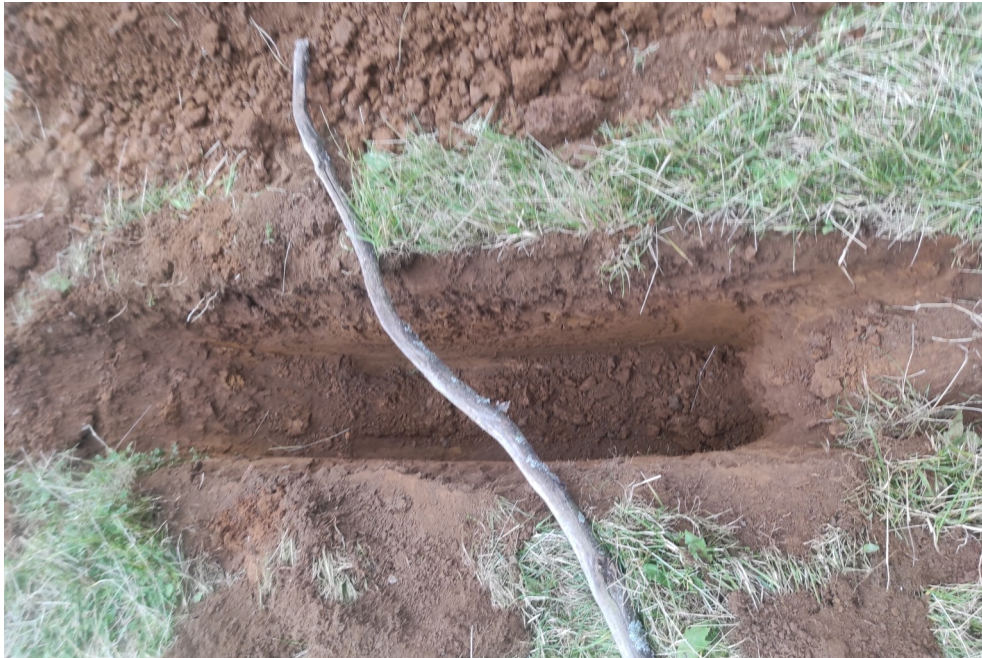
Photograph of trial pit SA8.
