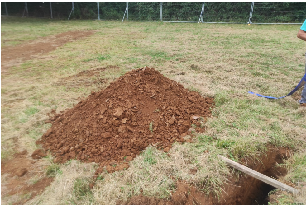
Photograph of arisings from trial pit SA5.
