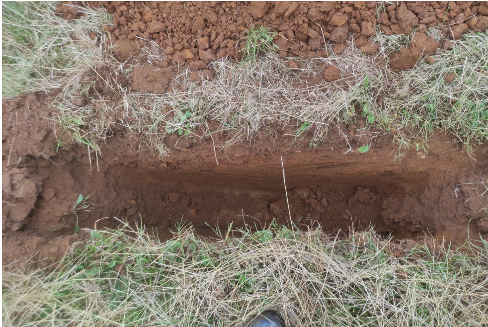
Photograph of trial pit SA2.
