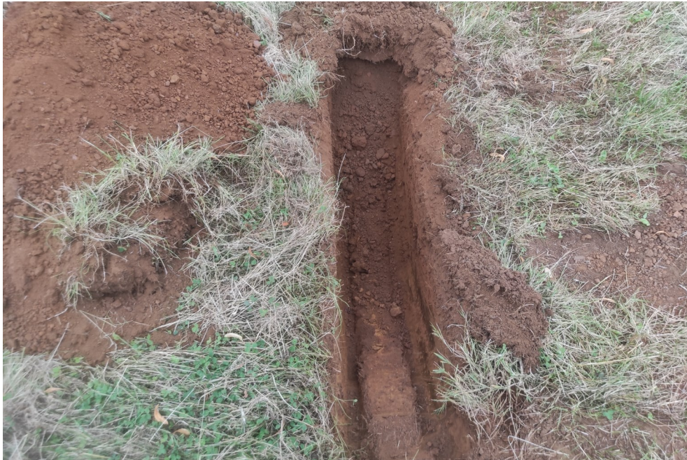
Photograph of trial pit SA7.
