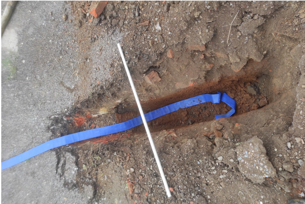
Photograph of trial pit SA1.
