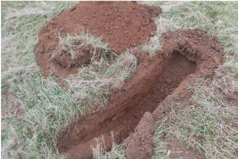
Photograph of arisings from trial pit SA7.
