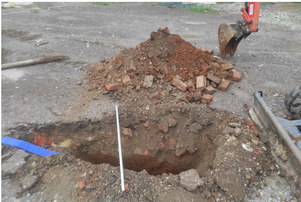
Photograph of arisings from trial pit SA1.
