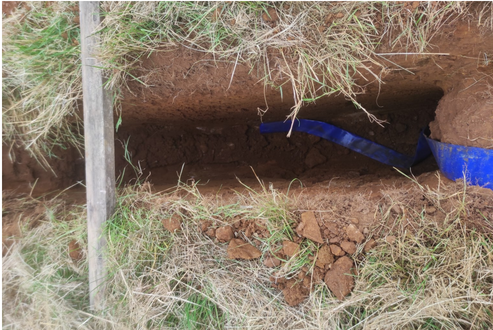
Photograph of trial pit SA4.
