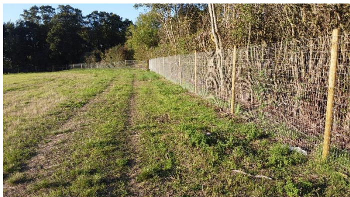
1.3.1 Typical fence detail (50mmx100mm mesh x2m high)
