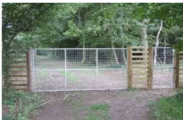
1.3.2 Vehicular gate detail (3.65m wide galvanised 40mm box frame and mesh), and pedestrian gate (1.2m wide)
