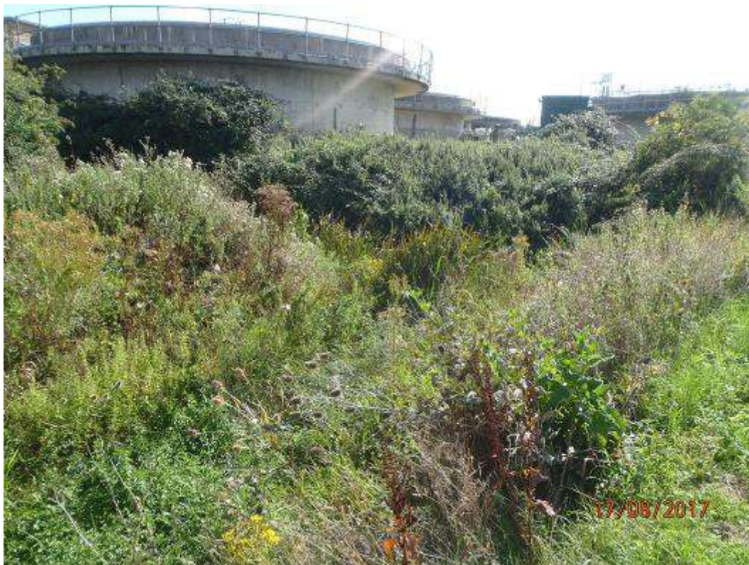
Photo 6— Drainage ditch to the east of site
