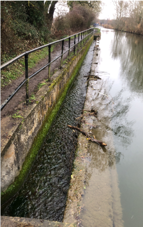
Figure 2.3: Side spill at Kidlington Green Lock
