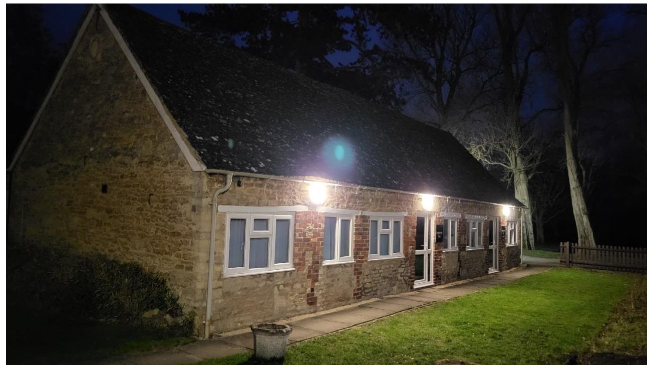
Figure 2.7– View 3, South – Begbroke farmhouse.
