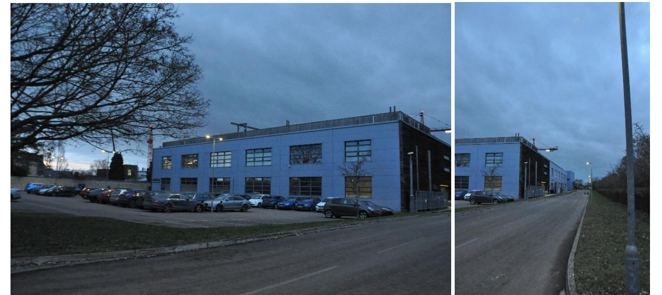
Figure 2.9 – View 5, Northwest – External car park and access roadway.
