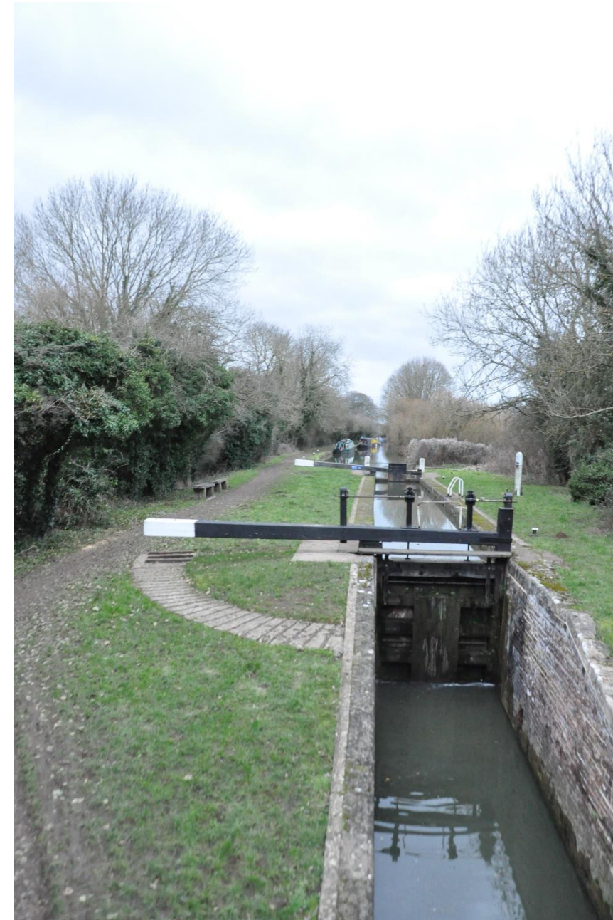
Figure 2.22 – View 18, South – Roundham Lock.
