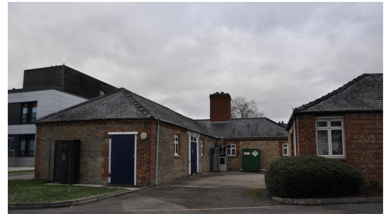
Figure 2.5 – View 1, North – Begbroke farmhouse.
