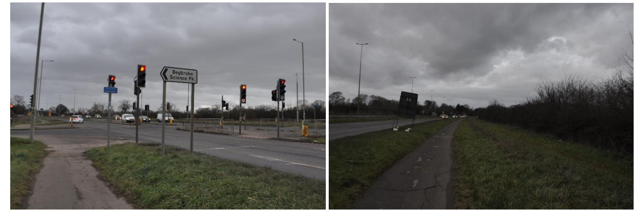
Figure 2.17 – View 12, South and North – A44
