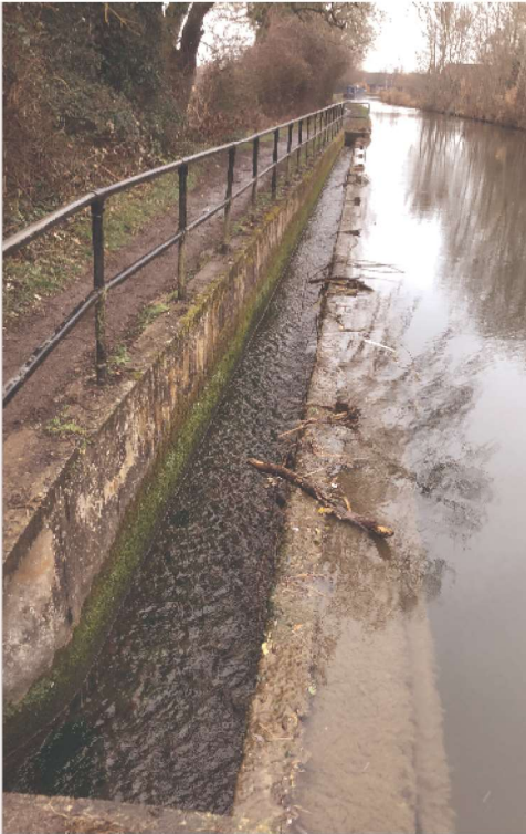
Figure 2.3: Side spill at Kidlington Green Lock
