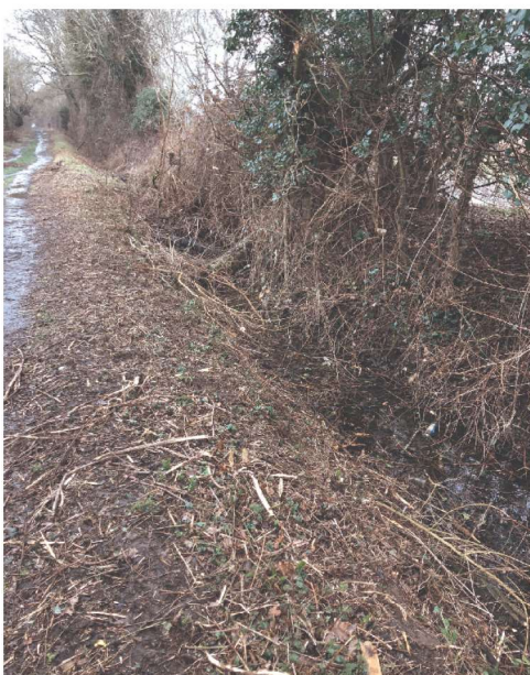
Figure 4.5: Example of the condition of the ditches running parallel to Yarnton/Green Lane
