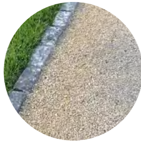
Light aggregate asphalt with cobble edging
