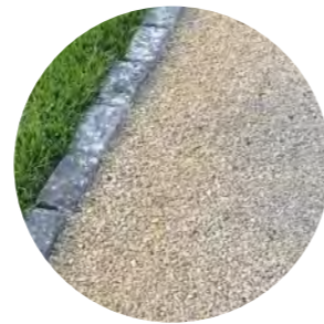
Light aggregate asphalt with cobble edging
