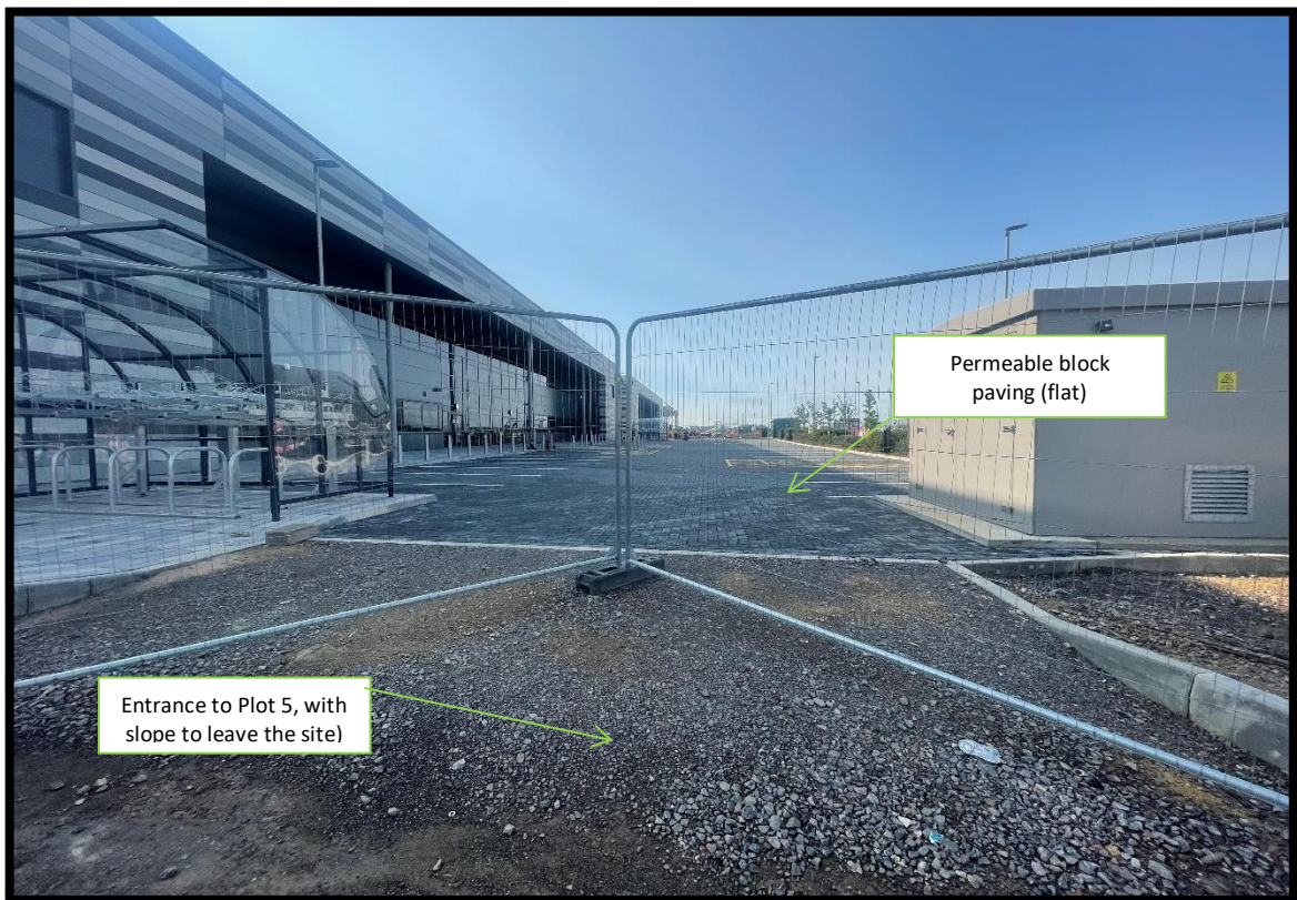
Fig. 3.6.3- Entrance from West to Plot 5
