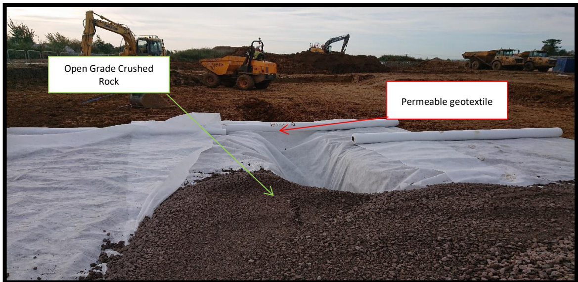
Fig 3.4.1- Filter trench construction with permeable geotextile and OGCR backfill.
