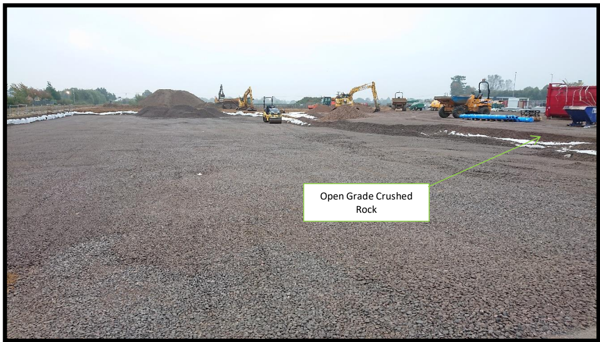
Fig 3.3.3- OGCR layer being compacted.
