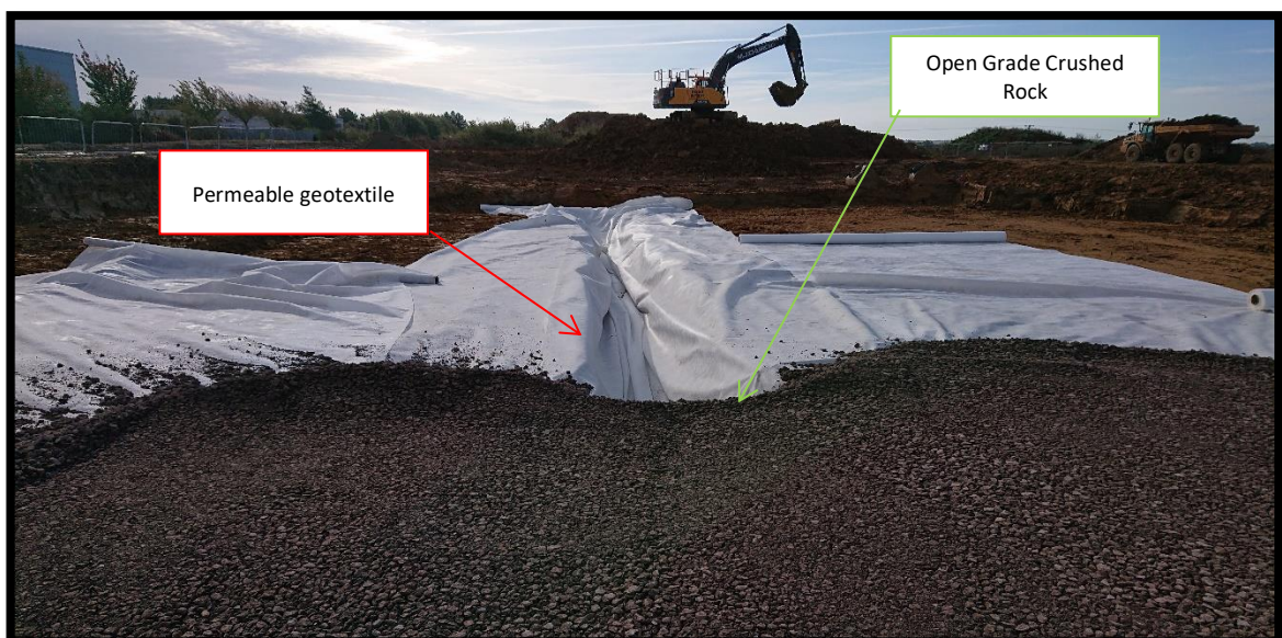
Fig 3.4.2- Filter trench construction with permeable geotextile and OGCR backfill.
