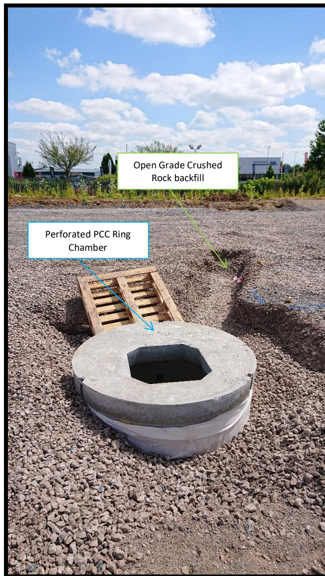
Fig 3.5.2- Perforated ring catch pit
