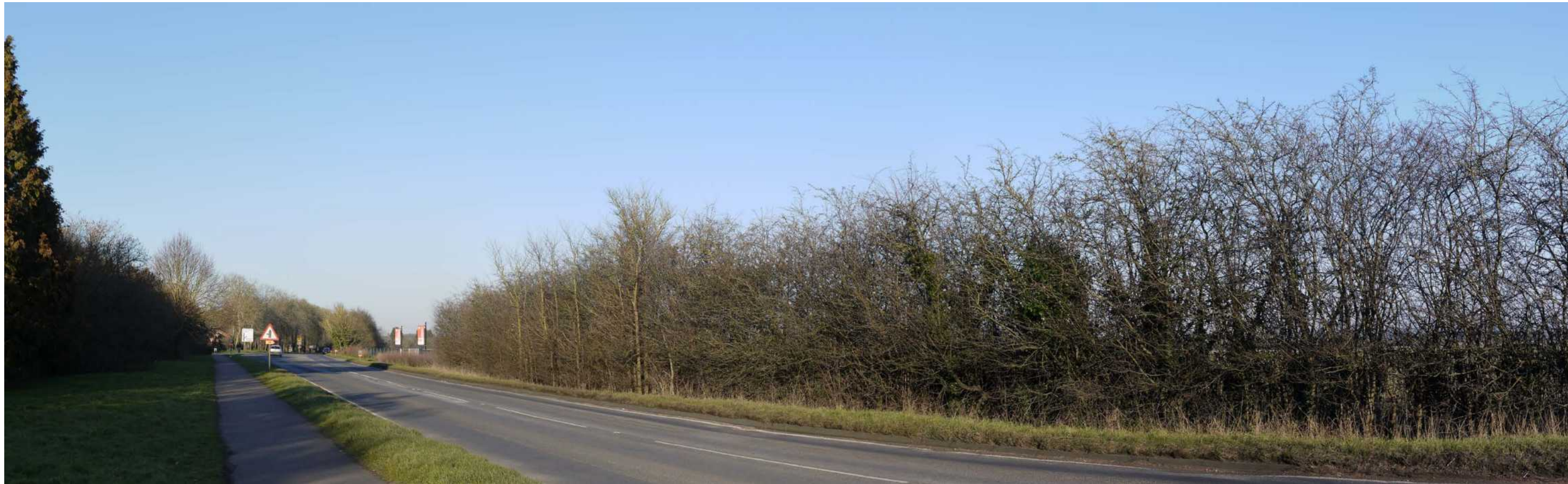
VP23 View from A4421 Roadside looking North towards Thompson Drive & East to Airfield
