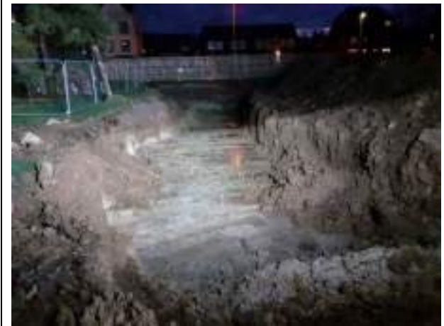
05.12.22 – Cell 3: Excavation progressed northwards with contaminated soils removed down to clean clays; contamination indicators absent along eastern and northern sidewalls.
