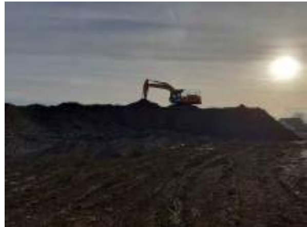
23.01.23 – Stockpiling of site-generated aggregate in south of site.
