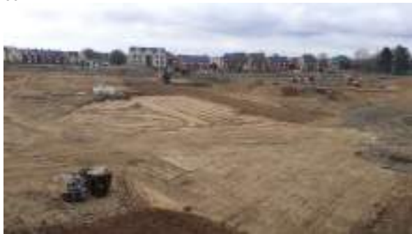
07.03.23 – View south across central part of site.
