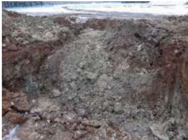
13.12.22 – Cell 7: Excavation and replacement of soils to east of Cell 7 Hotspot.
