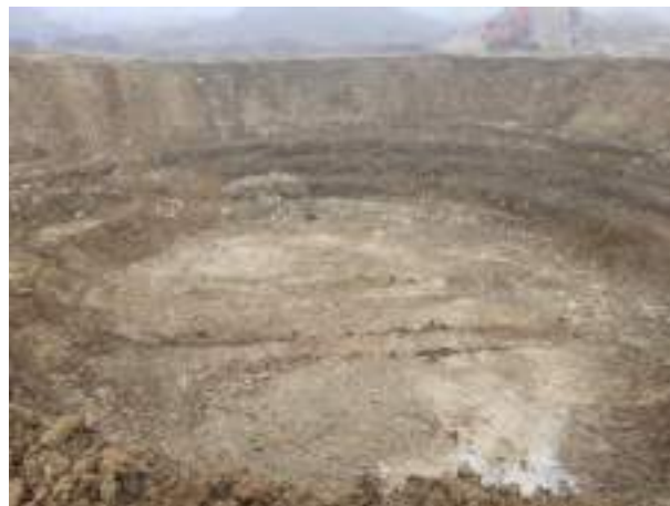
14.11.22 – View north across POL21A area following breakout and removal of tank.
