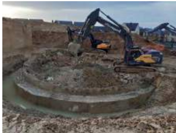
24.11.22 – Exposure of tank base
