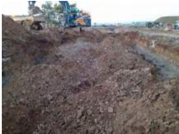
30.01.23 – Cell 2: Clean overburden soils replaced into excavation area.
