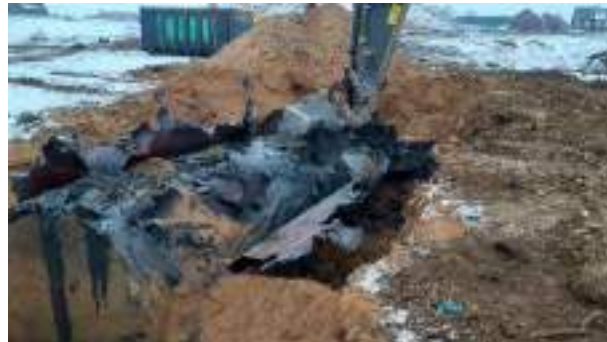
12.12.22 – Excavation of PFA from tank.
