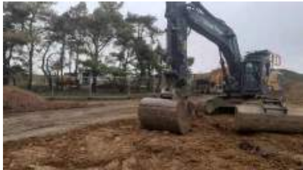
16.02.23 – Cell 9: Commencement of excavation from northwest extent of Cell 3
