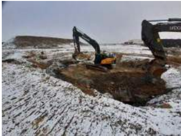
14.12.22 – Exposure of concrete slab overlying POL2 (North) tanks
