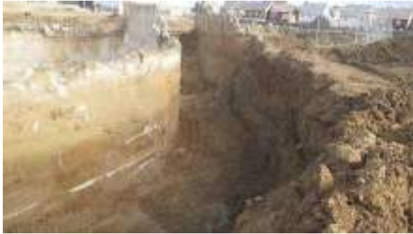
22.11.22 – POL21C tank walls fully exposed
