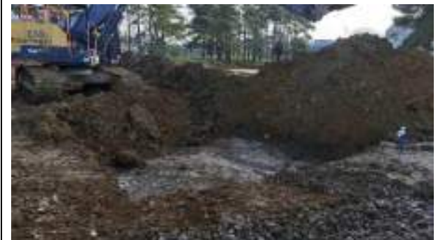
08.12.22 – Cell 6: Commencement of excavation to north of western part of Cell 4.
