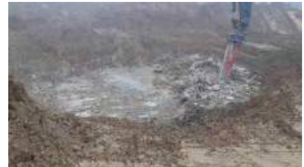
01.12.22 – Breakout of tank base.
