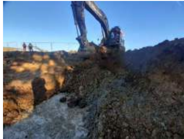
06.02.23 – Cell 5: Commencement of excavation from southwest extent of Cell 4.
