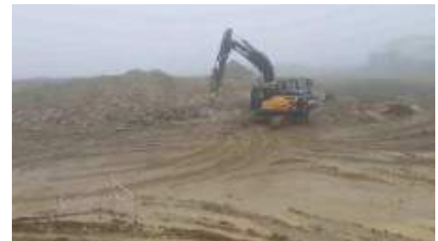
01.12.22 – Stockpile of recovered concrete undergoing further breaking to recover rebar.
