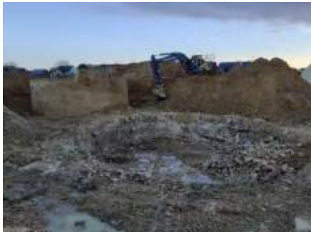
23.11.22 – Tank sidewalls demolished
