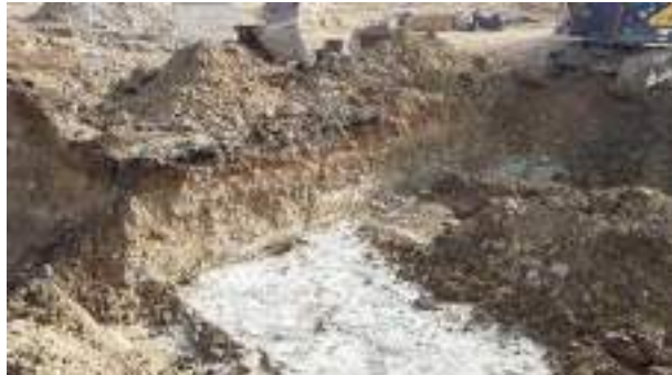
02.03.23 – No contamination indicators present along eastern sidewall as excavation progressed southwards.
