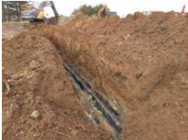
15.03.23 – Cell 10: Relict POL pipeline discovered to north of Cell 9 (1/2).
