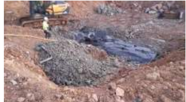
07.12.22 – Exposure of northernmost tank surrounded by PFA fill.
