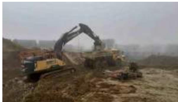
01.12.22 – Removal of broken out concrete to be stockpiled for processing.
