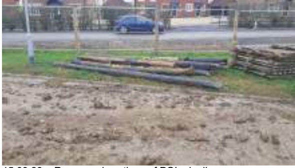
15.03.23 – Recovered sections of POL pipeline.
