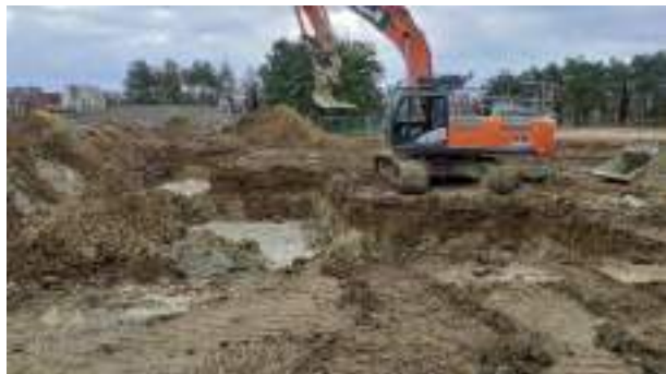
01.02.23 – Cell 3: View of entire Cell 3 excavation area.
