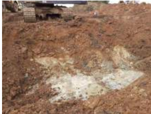
20.03.23 – Cell 10: Excavation progressed westwards; significant contamination indicators absent from western sidewall.
