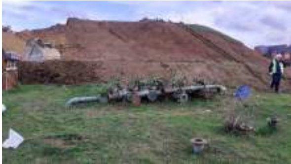
25.10.22 – Turf stripped from POL21 bund.
