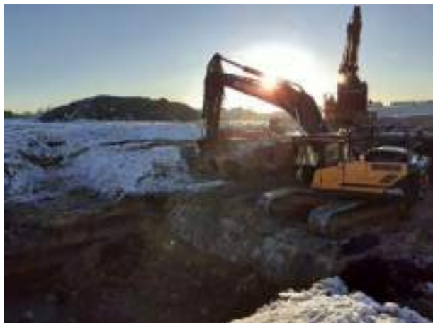
15.12.22 – Removal of broken out concrete slab and exposure of underlying tanks.
