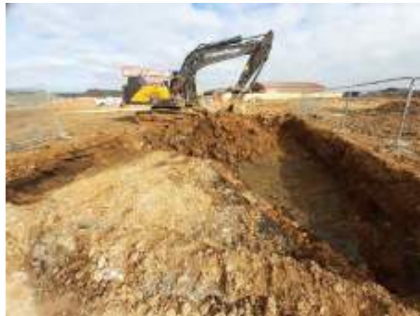
03.04.23 – Excavation of ACM impacted soils complete.
