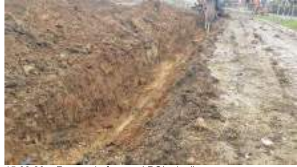
15.03.23 – Removal of second POL pipeline.
