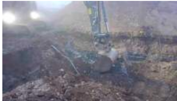
25.01.23 – Excavation of impacted soils progressed to west.
