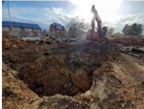
21.03.23 – Cell 11: Excavation complete and clean overburden soils replaced into excavation area.
