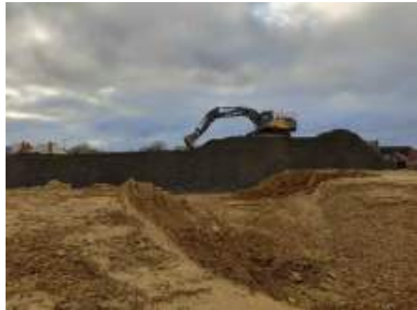
30.01.23 – Reprofiling of aggregate stockpile in southeast of site (stockpile ref: 'Agg-SP1').
