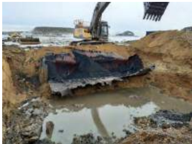
13.12.22 – Excavation of final tank and PFA from POL2 (South) area.
