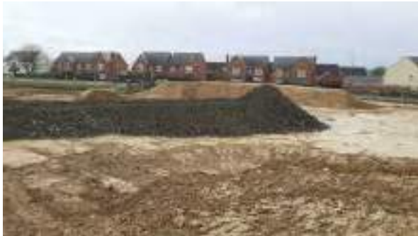
11.01.23 – Stockpiling of site-generated aggregate in south of site.
