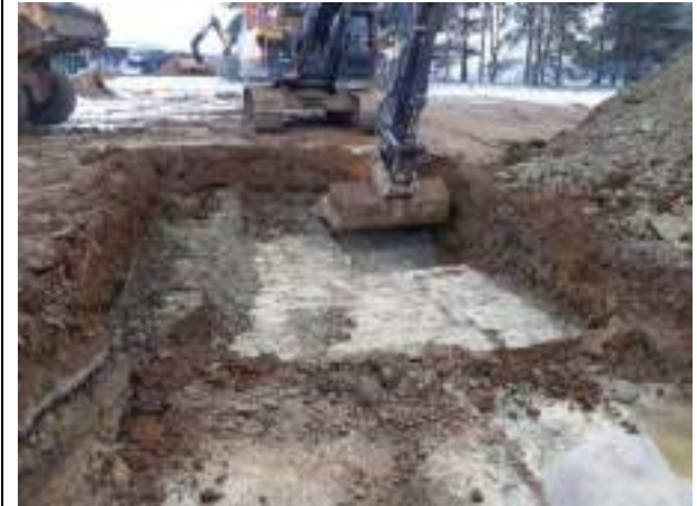
13.12.22 – Cell 7: Excavation of northern part of Cell 7 Hotspot.
