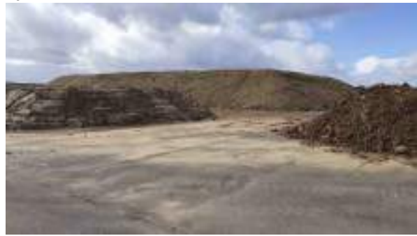
24.03.23 – Stockpiles of contaminated soils located within holding area in wider Heyford development site (4/5).
