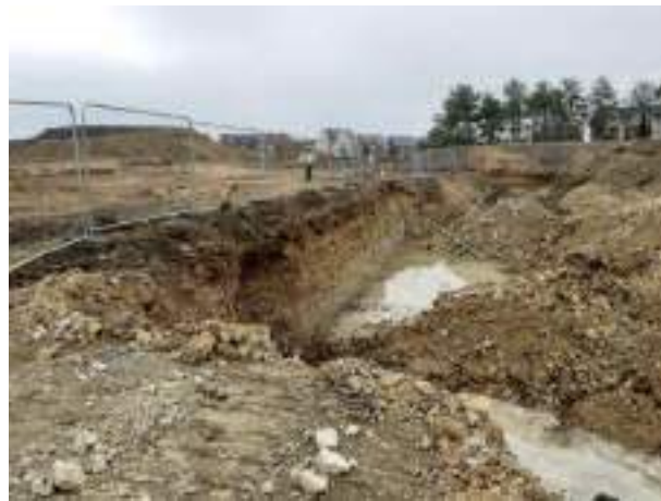
13.02.23 – Cell 7: View south along eastern sidewall.
