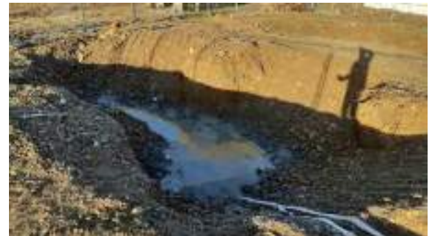
08.12.22 – Northernmost tank removed.
