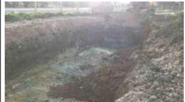
22.03.23 – Cell 12: Excavation progressed westwards with contaminated soils removed down to clean clays; contamination indicators present in southern sidewall but unable to progress due to standoff from Camp Road / live services.
