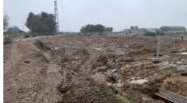
08.03.23 – Topsoil strip complete in centre-south / southwest of site following tree felling.
