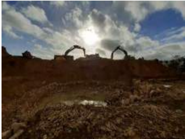
08.11.22 – POL21A tank walls broken out leaving concrete base exposed.
