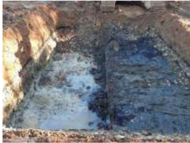
06.12.22 – Cell 4: Soils demonstrating slight contamination indicators but not significant enough to warrant removal so excavated, aerated and replaced into excavation.
