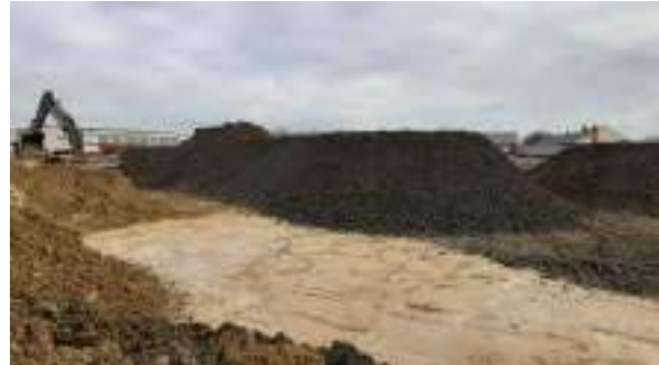
27.01.23 – Aggregate stockpile in southeast of site (stockpile ref: 'Agg-SP1').
