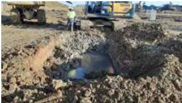
19.01.22 – Excavation of brick chamber in centre-northwest.
