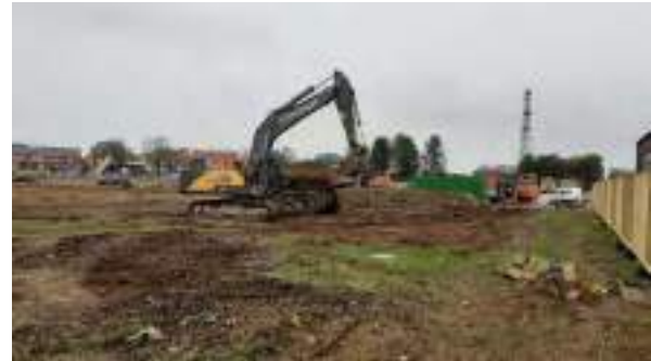
07.03.23 – Topsoil strip in north of site following tree felling (2/2).
