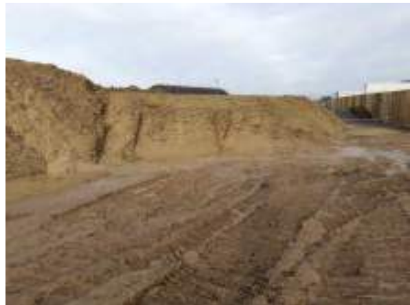
24.11.22 – Stockpile of hydrocarbon contaminated soils located on hardstanding in northwest of site.
