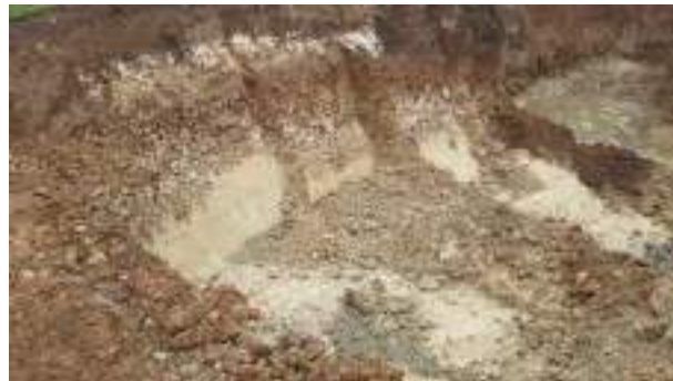
21.02.23 – No contamination indicators along northern extent of initial excavation area.
