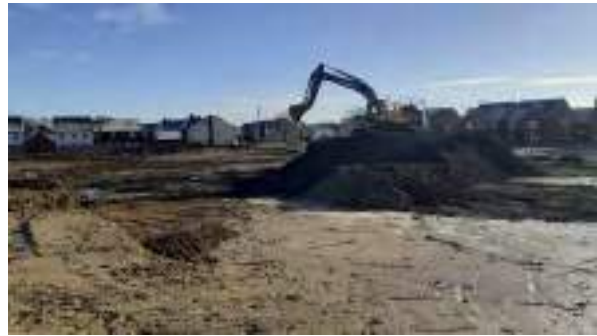
19.01.22 – Stockpiling of site-generated aggregate in south of site.
