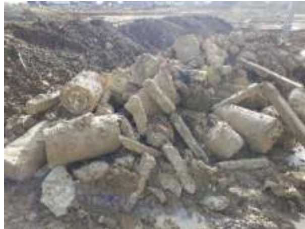
03.04.23 – Drums and posts excavated and removed.
