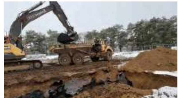
12.12.22 – Removal of PFA to hardcore stockpile.
