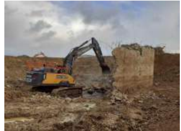
23.11.22 – Demolition of tank sidewalls
