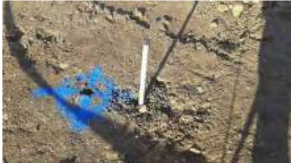
26.01.22 – Vapour probe (VP1) installation - West (2/2)
