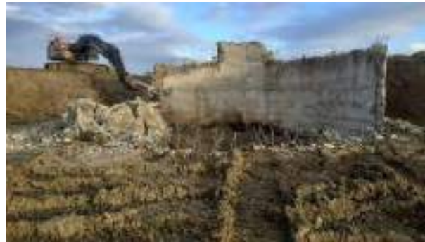
22.11.22 – Demolition of tank sidewalls
