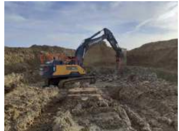
24.11.22 – Breakout of tank base
