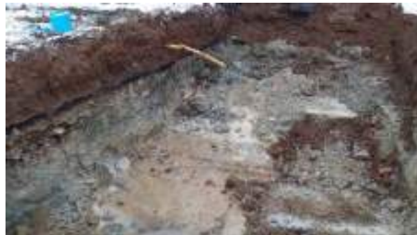
12.12.22 – Cell 7: Excavation of Cell 7 Hotspot progressed eastwards; contamination indicators absent from base and western / southern / eastern sidewalls but still present in northern sidewall (1/2).
