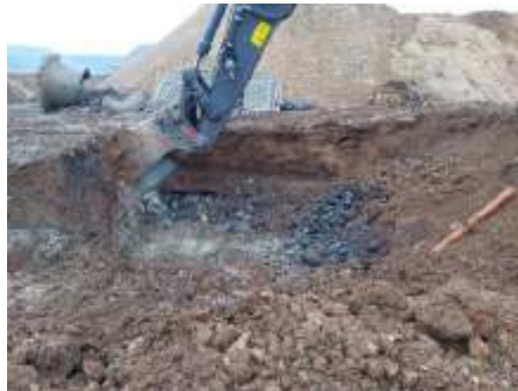
25.01.23 – Excavation of impacted soils to north of previous excavation area.
