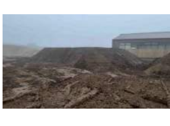
01.12.22 – Recovered topsoil stockpiled in centre-northwest of site (stockpile ref: TSSP3).
