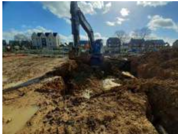
14.03.23 – Cell 9: Commencement of excavation from west of Cell 1 with removal of contaminated soils down to clean clays.
