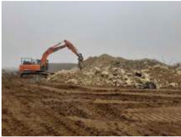
14.11.22 – Breaking of site won concrete to recover rebar.
