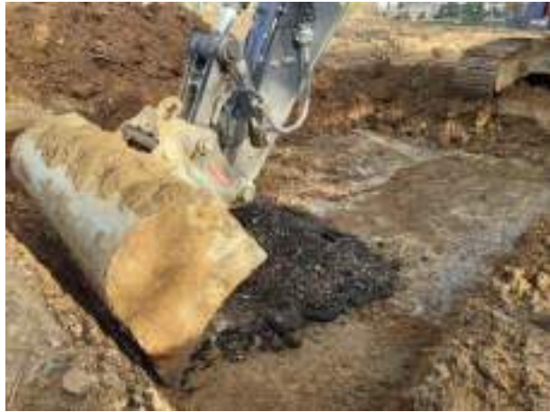
06.12.22 – Cell 4: Commencement of excavation (western extent of Cell 4).
