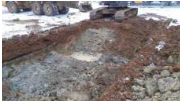
12.12.22 – Cell 7: Excavation and replacement of soils to east of Cell 7 Hotspot.
