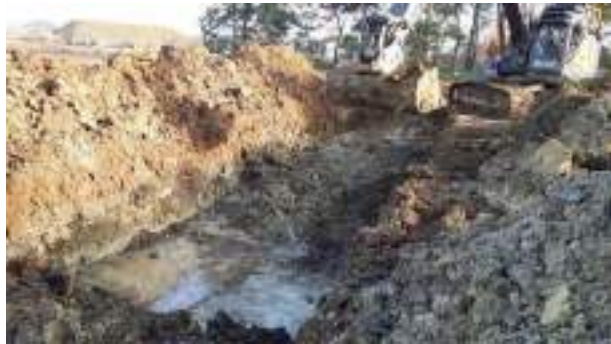
07.12.22 – Cell 5: Excavation and replacement of soils progressed eastwards.
