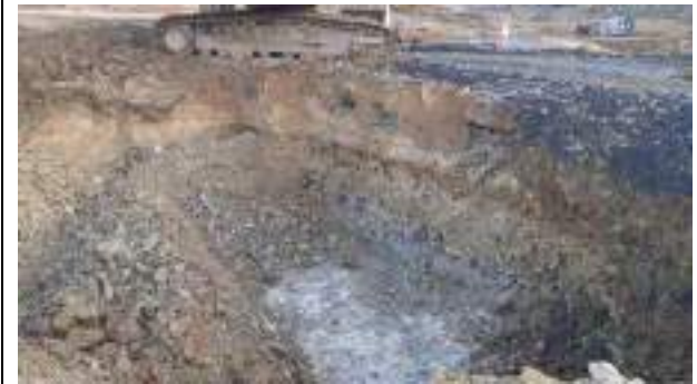
10.02.23 – Cell 7: Excavation progressed northwards with contaminated soils removed down to bedrock; significant contamination indicators absent along eastern sidewall.
