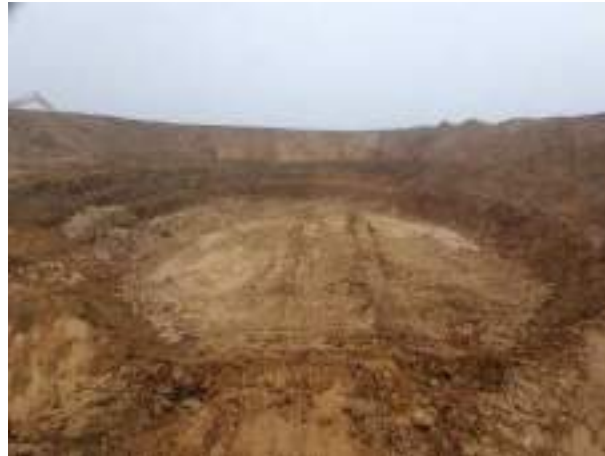
14.11.22 – View west across POL21A area following breakout and removal of tank.
