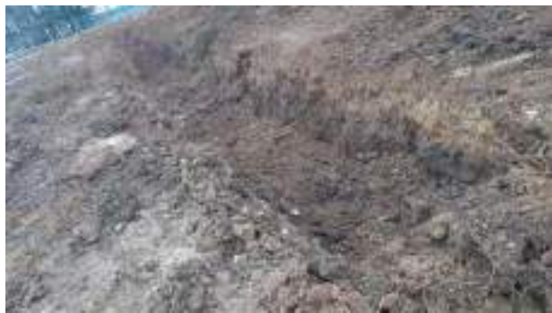
15.03.23 – Cell 10: Soil placed into trench to soak up leaked jet fuel – to be removed at later date.
