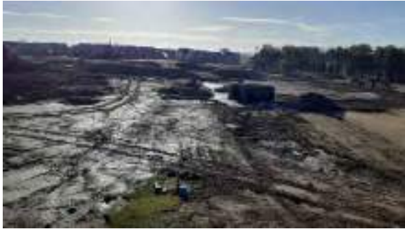
19.01.22 – View south across central part of site.
