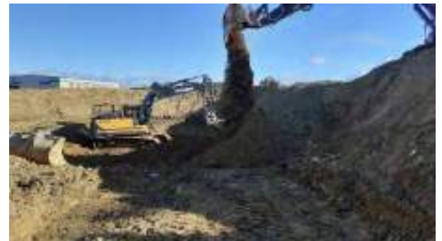
18.11.22 – Backfilling of POL21A area with site recovered soils.
