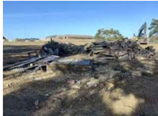
18.10.22 – Interceptor demolition arisings and valve pit in centre-southwest of site.
