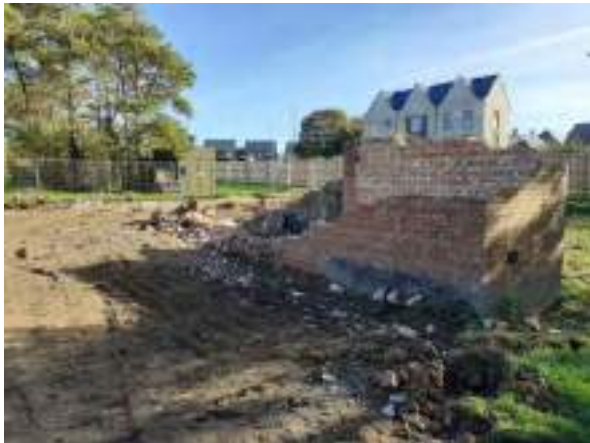
18.10.22 – Partially demolished interceptor in centre-southwest of site.
