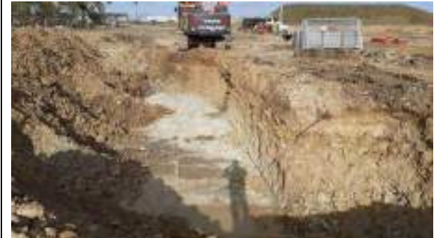
09.02.23 – Cell 6: View of entire Cell 6 excavation area.
