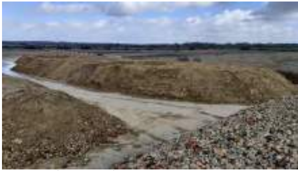
24.03.23 – Stockpiles of contaminated soils located within holding area in wider Heyford development site (1/5).
