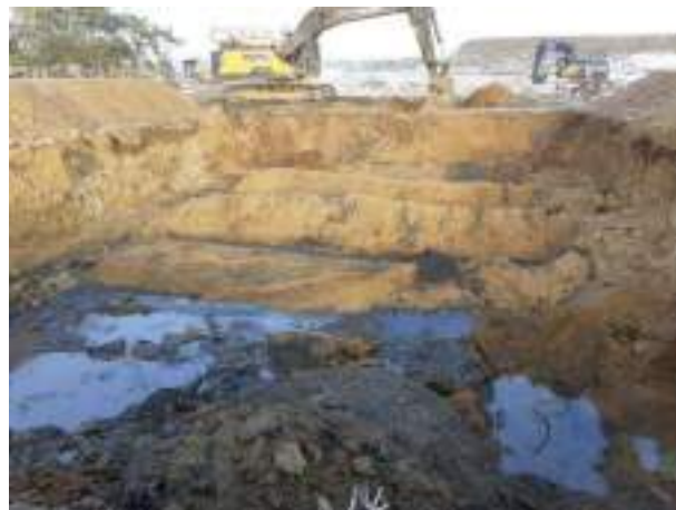
14.12.22 – View north across POL2 (South) area following tank removal.
