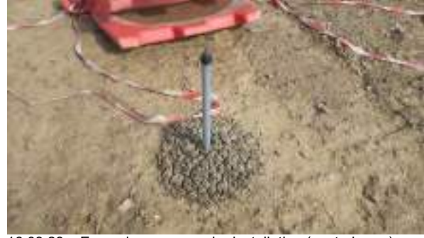
16.03.23 – Example vapour probe installation (central area)
