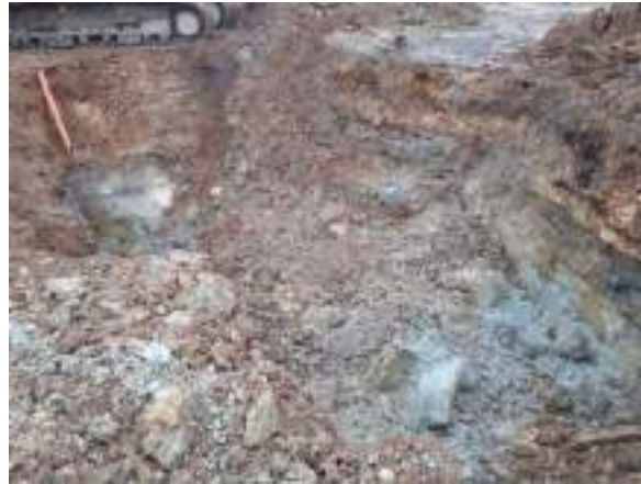
25.01.23 – Relict interceptor tank and associated pipework removed.
