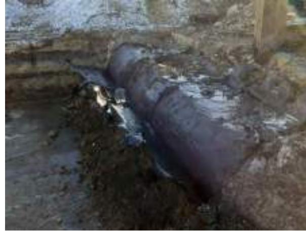
15.12.22 – Tank opened exposing PFA fill.
