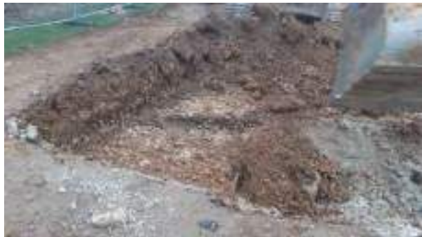
16.02.23 – Cell 9: Excavation progressed to north of previous excavation area.
