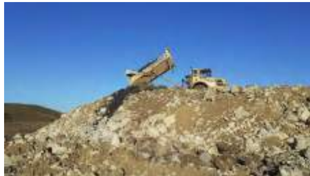
08.12.22 –PFA tank fill relocated to hard materials stockpile.
