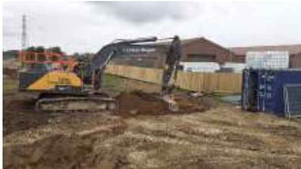
07.03.23 – Topsoil strip in north of site following tree felling (1/2).
