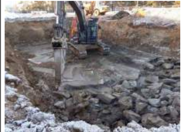
15.12.22 – Further breakout of concrete slab overlying POL2 (North) tanks.
