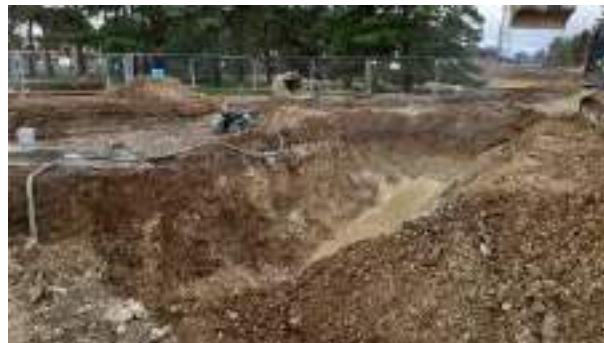
02.02.23 – Cell 4: Commencement of excavation from southern extent of Cell 3.
