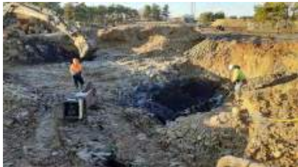
08.12.22 – Northernmost tank broken open and PFA fill excavated.
