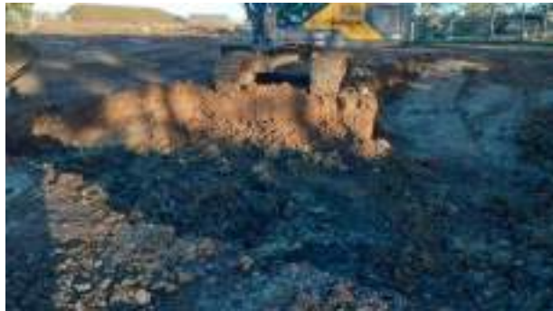
08.12.22 – Cell 7: Commencement of excavation to north of western part of Cell 6.
