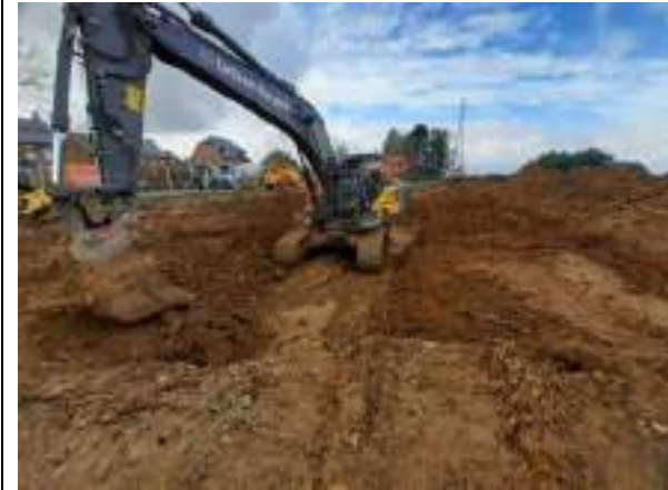
20.03.23 – Cell 10: Excavation complete and clean overburden soils replaced into excavation area.
