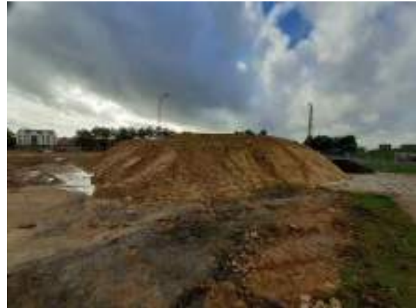
09.11.22 – Soils from POL21 tank excavations stockpiled on concrete hardstanding in northwest.
