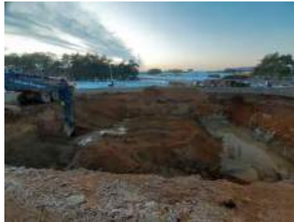
14.12.22 – Continued excavation of sands which separated tanks within POL2 (South) area.
