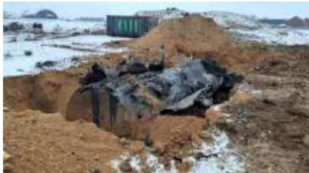
12.12.22 – Exposure of POL2 (South) tank.
