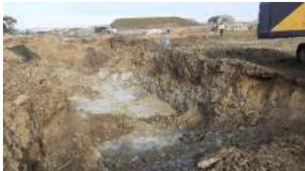
10.02.23 – Cell 7: View of entire Cell 7 excavation area.
