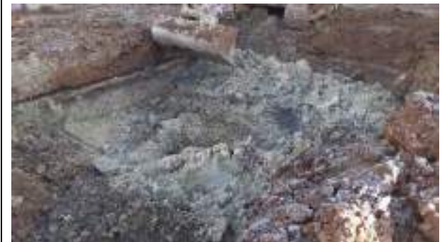
08.12.22 – Cell 6: Excavation and replacement of soils to east of Cell 6 Hotspot.
