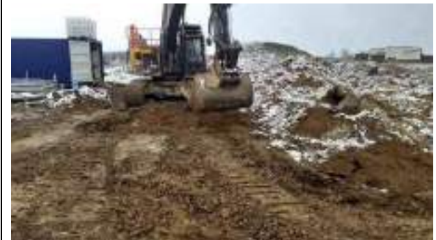
08.03.23 – Excavation continued to north of previous excavation area.
