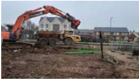
08.03.23 – Removal of relict cables in south of site.
