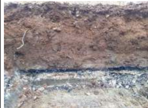
25.01.23 – Impacted soils present from layer of black, weathered asphalt into underlying silver clays.
