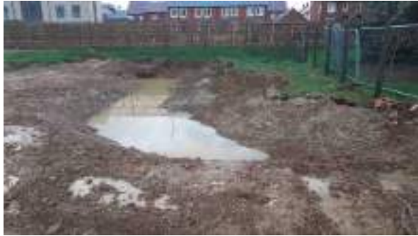
17.11.22 – Full demolition of interceptor in centre-southwest including breakout of floor slab.
