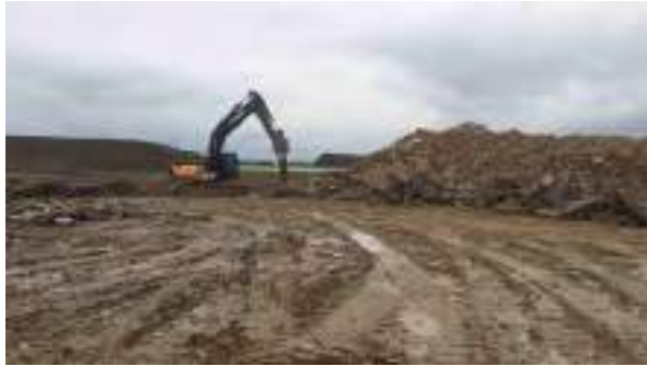
17.11.22 – Breaking of site won concrete to recover rebar.
