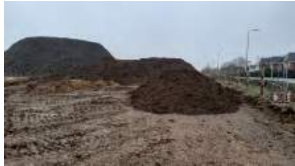
08.03.23 – Stripped topsoil stockpiled in southeast of site (stockpile ref: 'TS-SP5').
