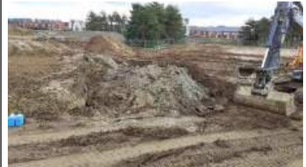
02.02.23 – Full excavation extent; excavation backfilled with clean overburden soils.
