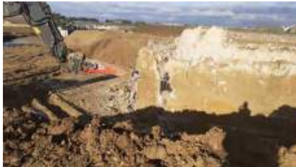
22.11.22 – Demolition of tank sidewalls
