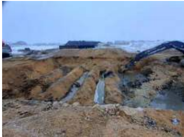
14.12.22 – Excavation of sands which separated tanks within POL2 (South) area
