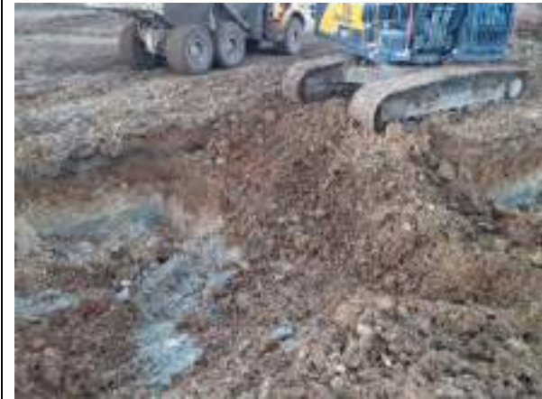
31.01.23 – Cell 2: Excavation progressed northwards with contaminated soils removed down to bedrock; significant contamination indicators absent along western sidewall.
