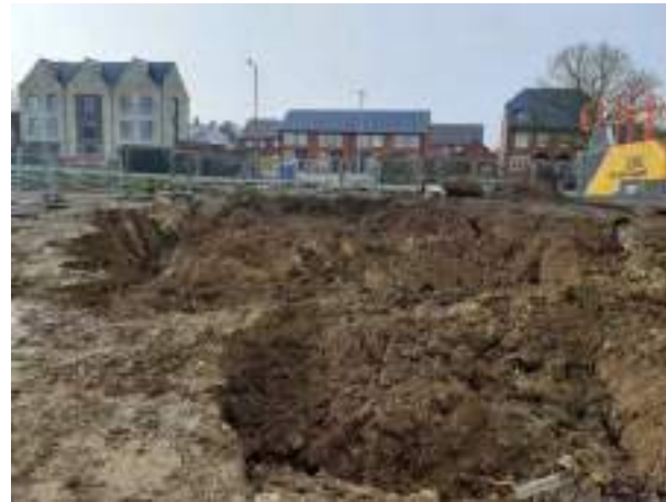
14.03.23 – Cell 9: View of Cell 9 excavation area (day 1).
