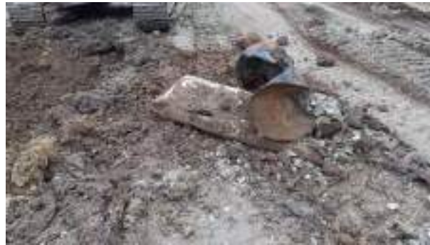
02.02.23 – Degraded metal drum removed from north of excavation area.
