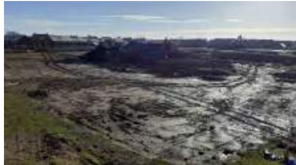
19.01.22 – View southeast across central part of site.
