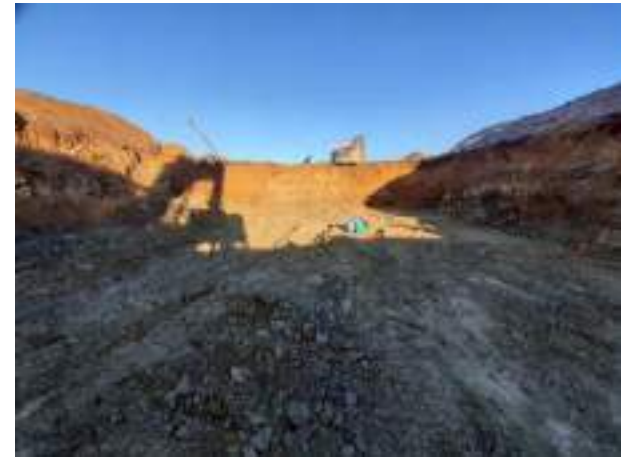
15.12.22 – Excavation of sands from POL2 (South) area complete and sidewalls exposed.
