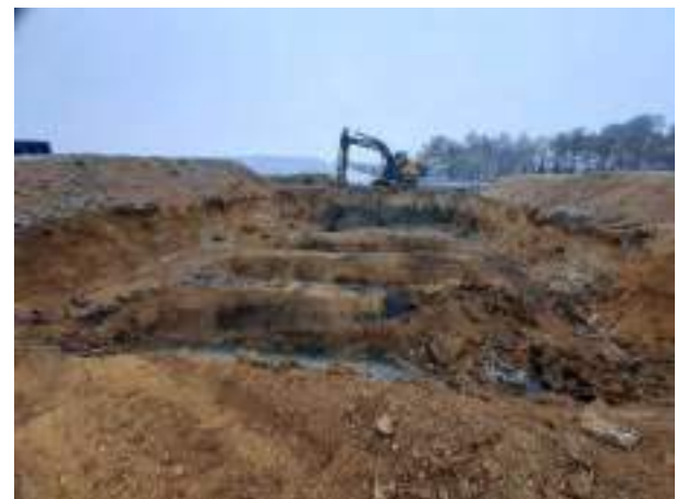
14.12.22 – View south across POL2 (South) area following tank removal.
