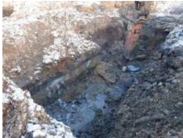
14.12.22 – Concrete base in area of northernmost tank undergoing breakout.
