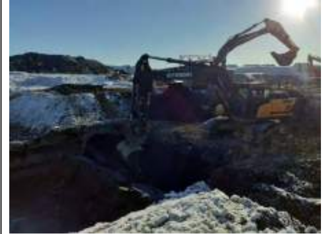
15.12.22 – Removal of PFA to hardcore stockpile.
