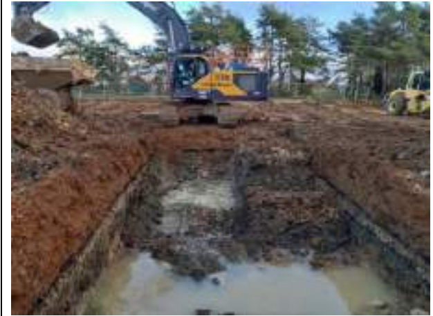
06.12.22 – Cell 4: Excavation and replacement of soils progressed eastwards
