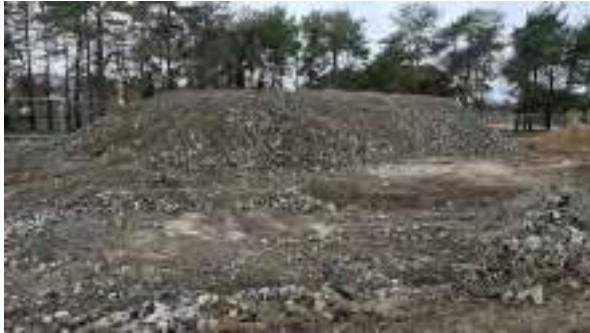
27.01.23 – Aggregate stockpile in south of site (stockpile ref: 'Agg-SP2').
