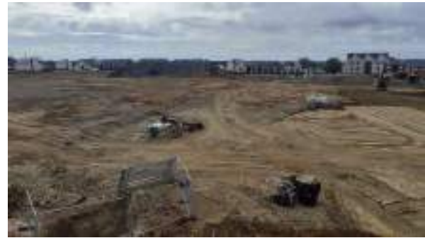
07.03.23 – View southeast across central part of site.
