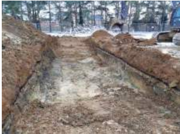
13.12.22 – Cell 8: Excavation progressed northwards; southern / northern extents of contamination hotspot identified.
