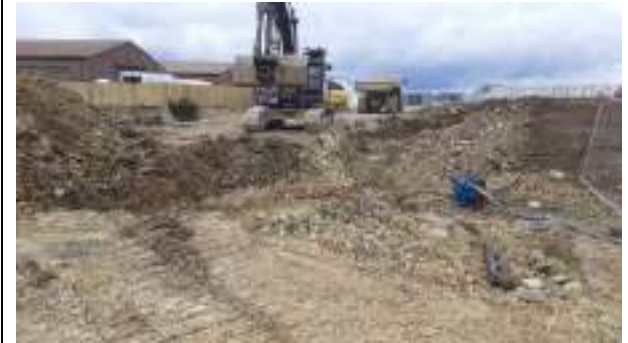
06.03.23 – Excavation continued to west of previous excavation area.
