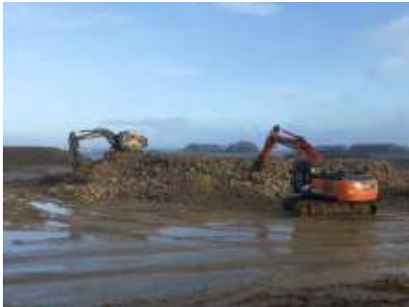
28.11.22 – Breaking of site won concrete to recover rebar.
