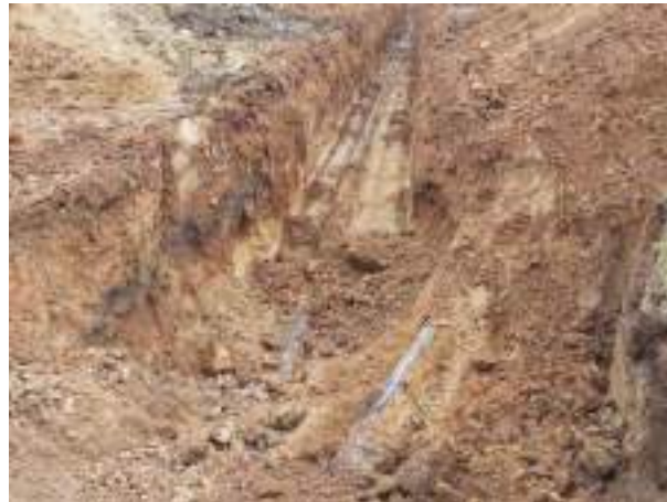
15.03.23 – Cell 10: Cell 10: Relict POL pipeline discovered to north of Cell 9 (2/2).
