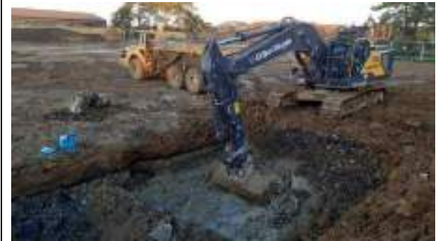
08.12.22 – Cell 6: Excavation of Cell 6 Hotspot down to clean clays.
