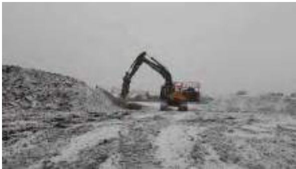
12.12.22 – Breaking of site won concrete to recover rebar.
