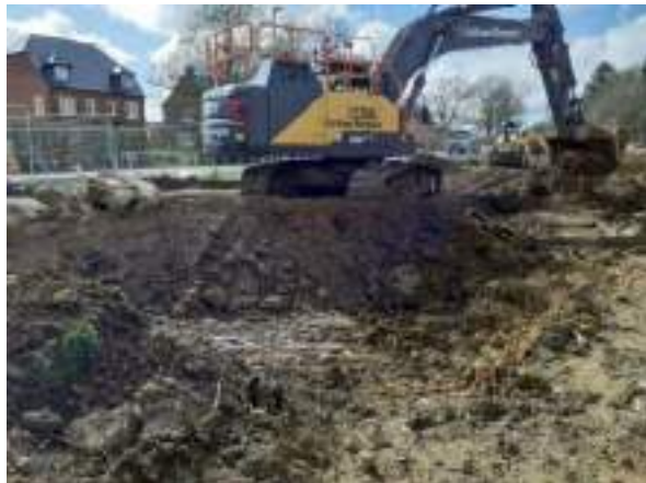
21.03.23 – Cell 11: Commencement of excavation from south of Cell 3.
