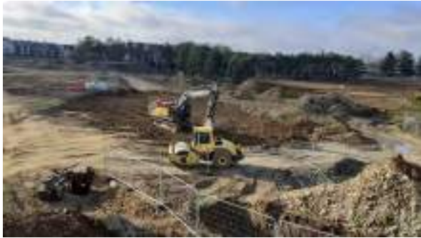
20.02.23 – Backfilling of 'Central Hotspot' excavation area with suitable site soils.
