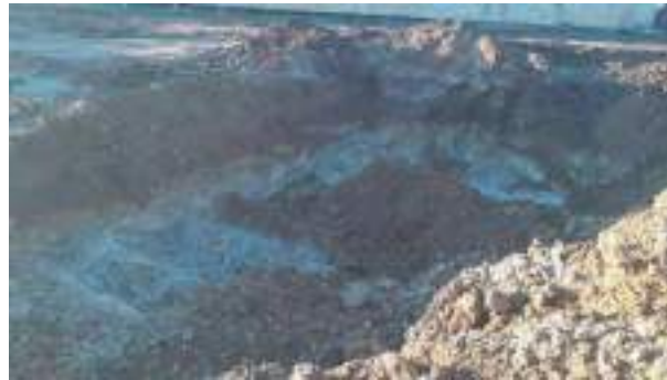
07.03.23 – Cell 9: Excavation progressed northwards / westwards with contaminated soils removed down to bedrock; significant contamination indicators absent along western and northern sidewalls.
