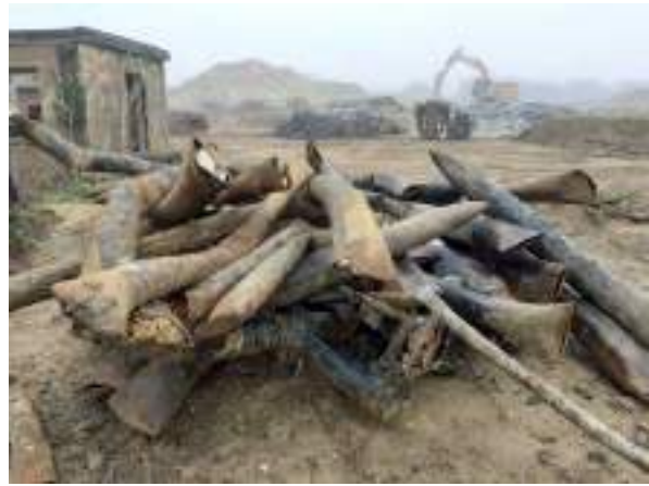
14.11.22 – Recovered sections of the decommissioned POL pipeline.
