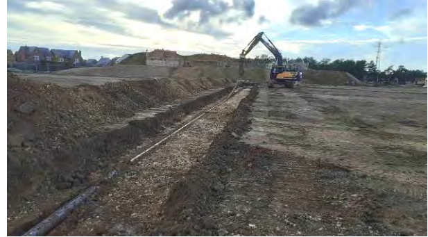
25.10.22 – Breakout of central / eastern sections of relict POL pipeline.
