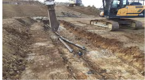
25.10.22 – Breakout of western section of relict POL pipeline.
