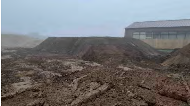
01.12.22 – Topsoil stockpile (TS-SP3)
