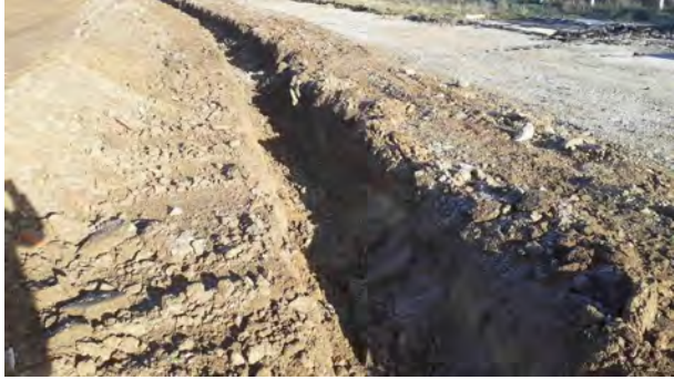
19.01.22 – ACM pipeline excavation (centre).
