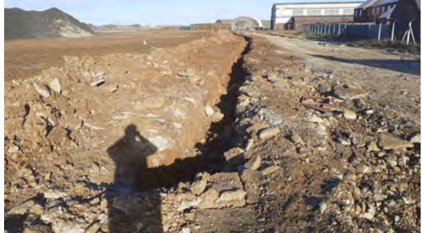
19.01.22 – ACM pipeline excavation (south).
