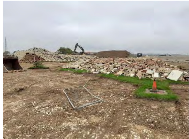
18.10.22 – Stockpiles of recovered hardstanding in northern part of site.
