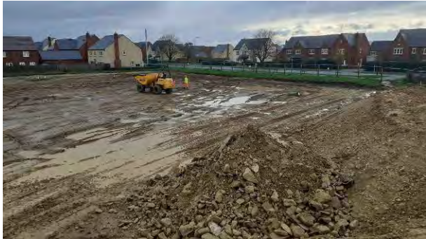
09.11.22 – Earthworks complete: view southeast across south of site.
