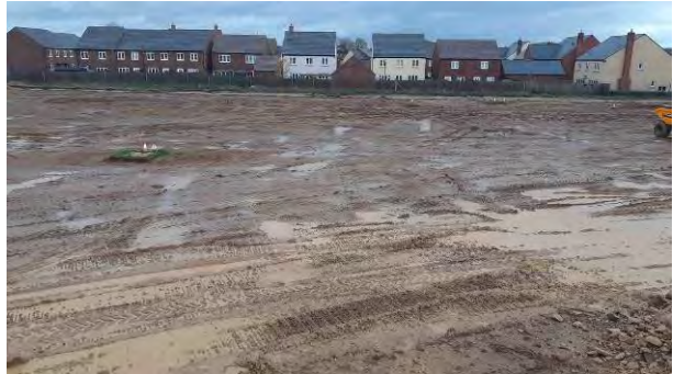
09.11.22 – Earthworks complete: view east across centre of site.
