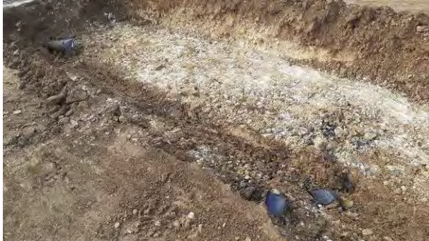
25.10.22 – No contamination indicators in soils underlying western section of relict POL pipeline (1/2).
