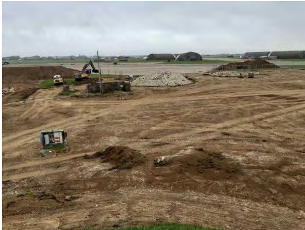
18.10.22 – View north across north / north-western part of site; stockpiles of site-recovered topsoil located offsite to north (TS-SP2) and northwest (TS-SP1) of site.
