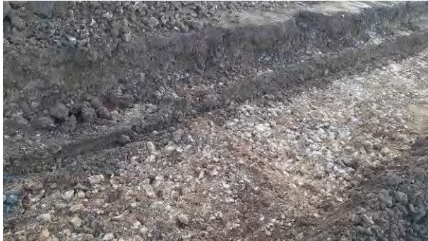
25.10.22 – No contamination indicators in soils underlying central section of relict POL pipeline.
