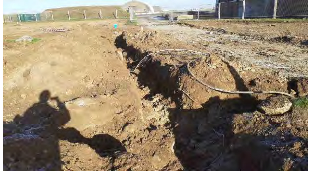
19.01.22 – ACM pipeline excavation (north).
